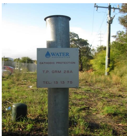
Cathodic protection test point (left); valve cover (right)
