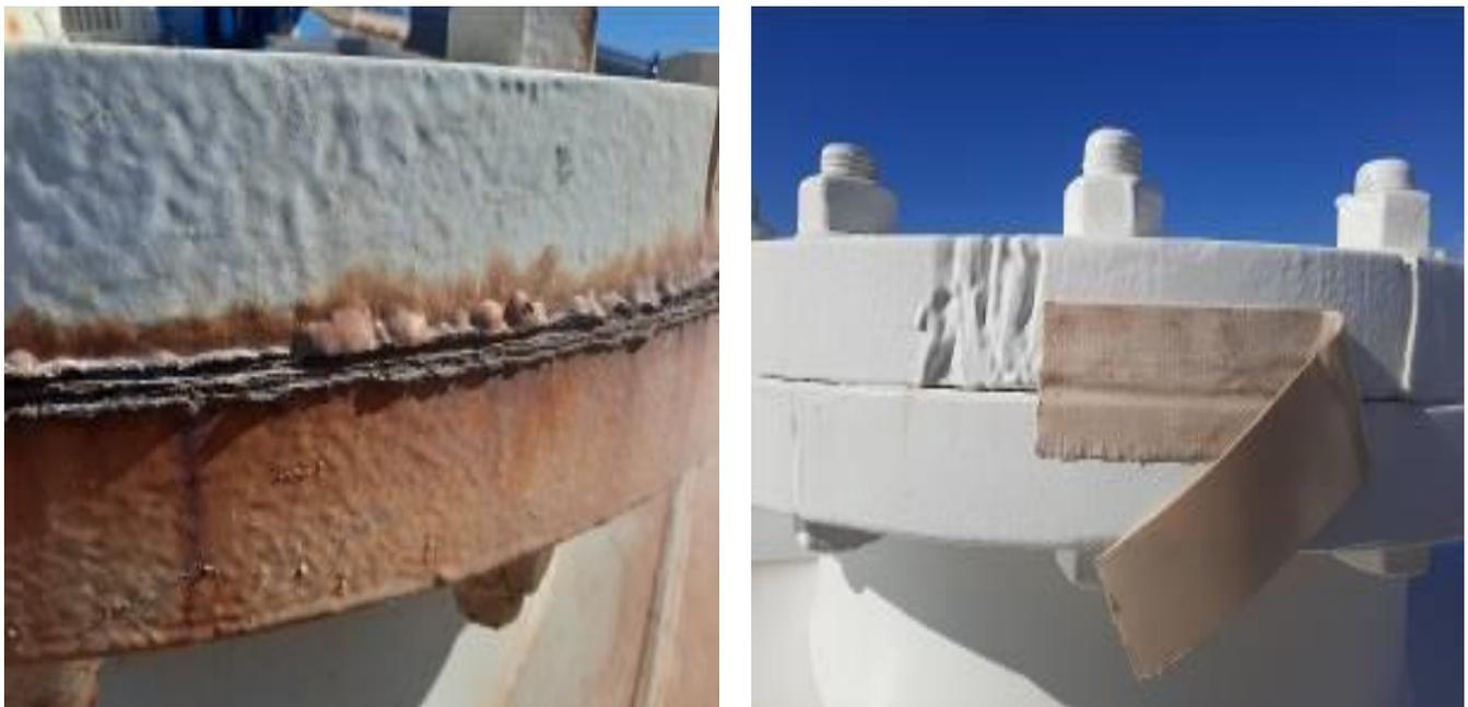
Photo 4. Visco-elastic tape application around a recoated flange is used to prevent under film corrosion and staining.
