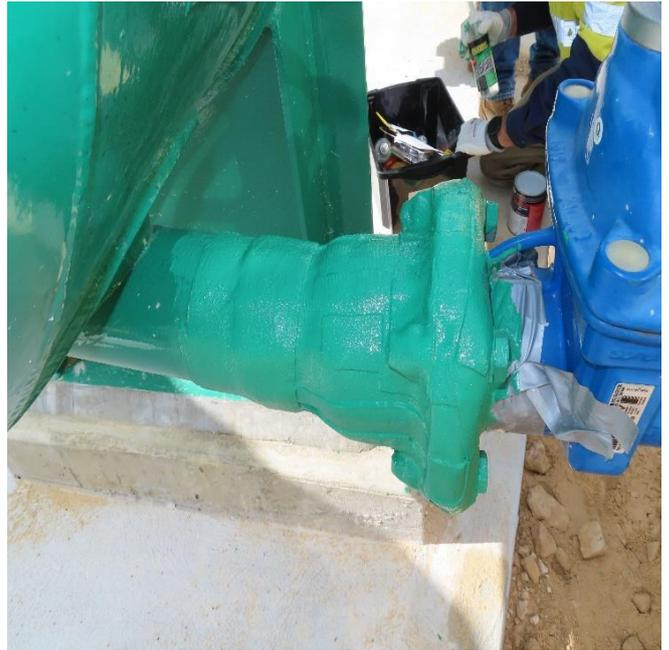
Photo 1. Above ground scour valve offtake before and after visco-elastic tape application.
