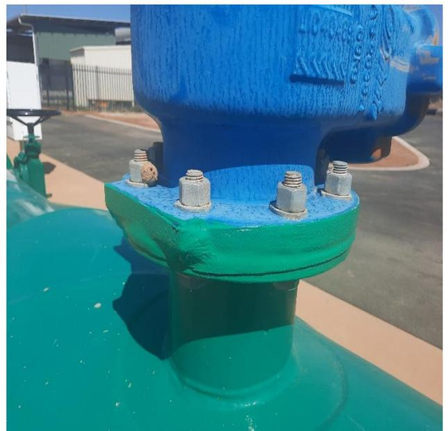
Photo 2. Visco-elastic tape application around coated flange circumference is used to prevent corrosion.
