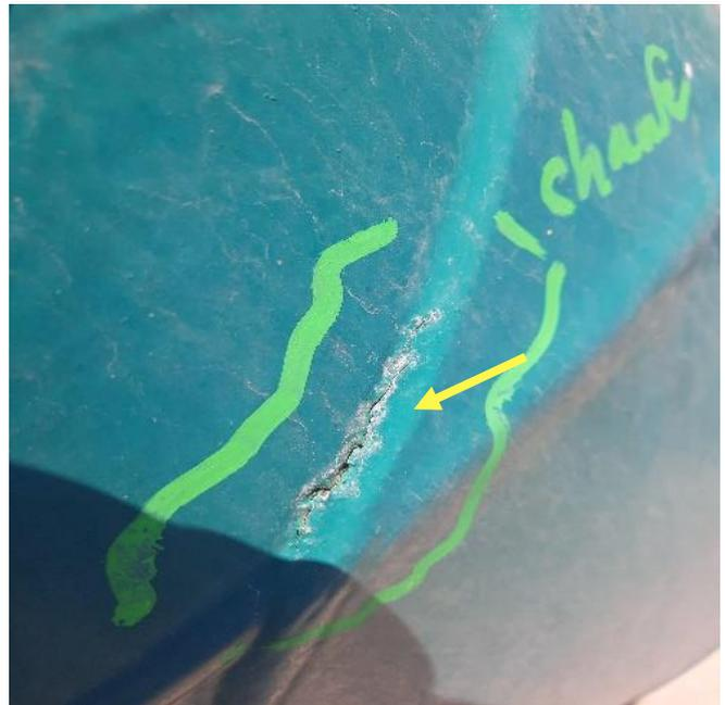
Photo 5. Visco-elastic tape application, where existing Sintakote termination has failed.
