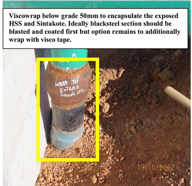
Photo 6. Visco-elastic tape is used on exposed heat shrink sleeve to provide UV protection and to prevent moisture ingress at HSS termination.
