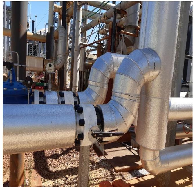
Photo 7. Thermal insulation is installed following completion of Visco-elastic Tape to all pipework and flanges to prevent corrosion under insulation
