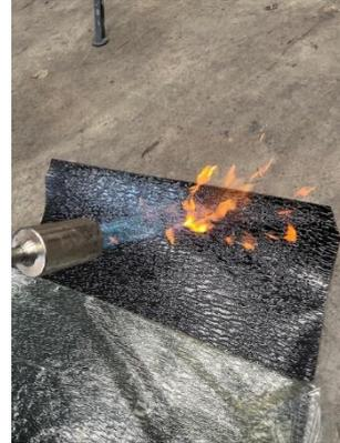
Pre-warm adhesive on sleeve leading edge to ensure good initial bond to steel and Sintakote.
