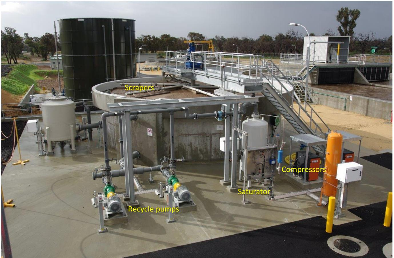
Figure 2-1: Image of thickening DAF showing DAF tank, scraper system, recycle pumps and saturator system
