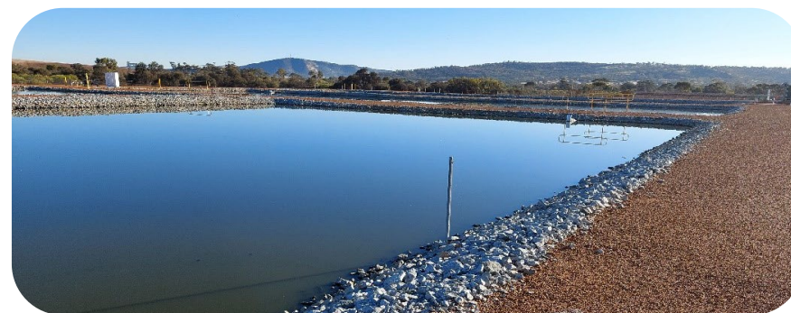
Figure 10: York WWTP primary pond
