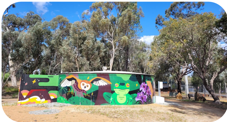
Figure 16: Wundowie water recycling tank
