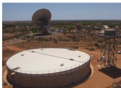
Sealed tanks and bores
