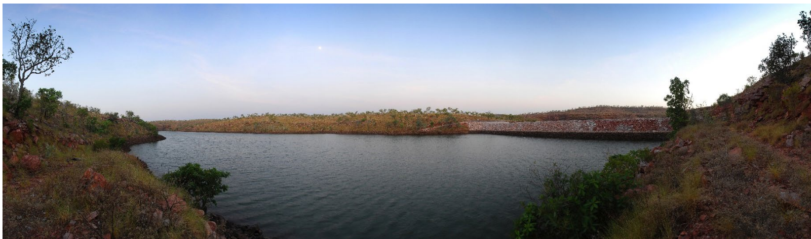
Figure 1: Moochalabra Dam - Wyndham
