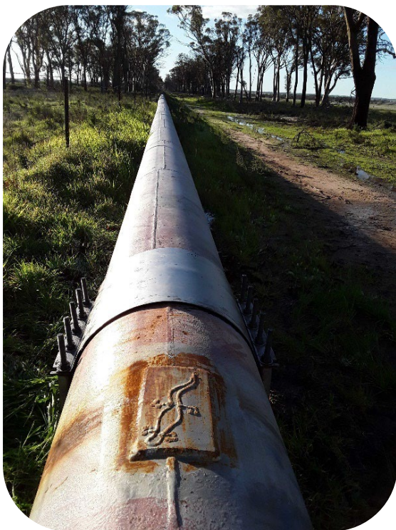
Figure 26: Section of the Goldfields pipeline
