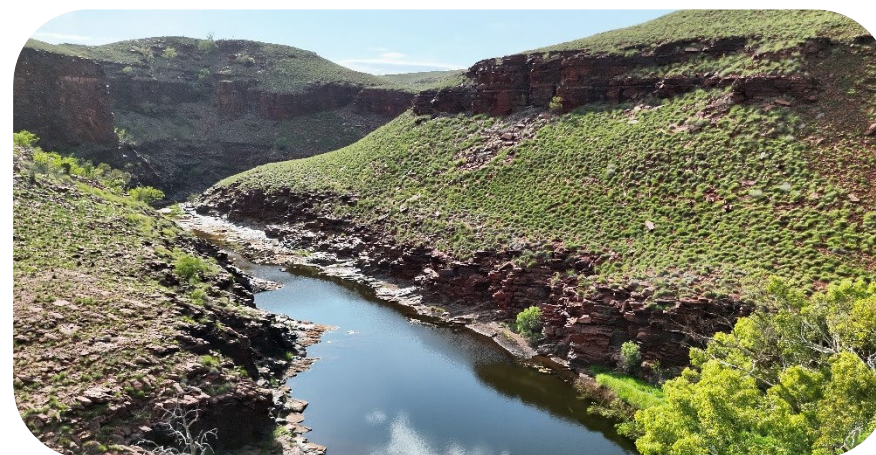
Figure 18: Harding Dam catchment (by drone)
