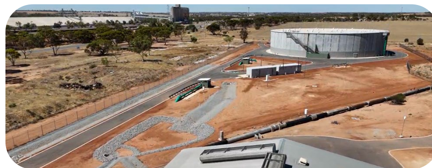
Figure 27: Merredin water tank
