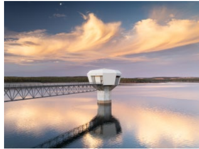
Large reservoirs with long detention times
