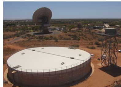
Sealed tanks and bores
