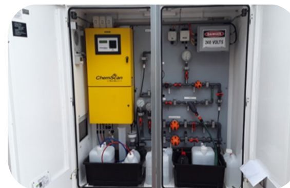
Figure 31: Advanced analyser installed on GAWS
