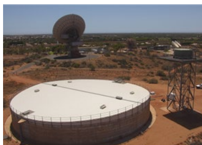
Sealed tanks and bores
