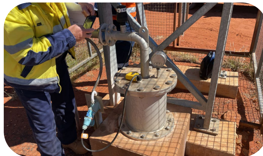
Figure 4: Thorough physical assessment of asset conditions informs improvement projects
