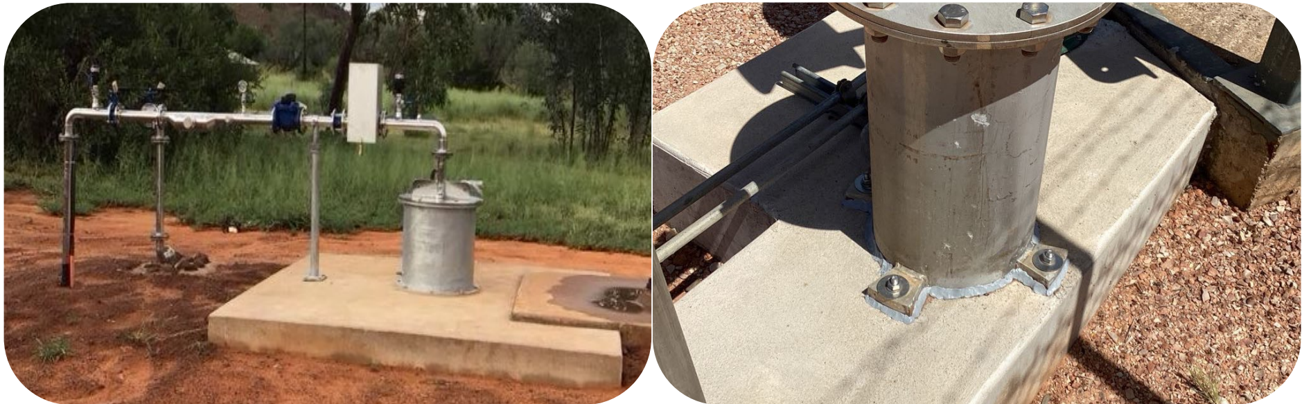
Figure 11: Bore sealing improved with upgrades to headworks and using sealants where possible
