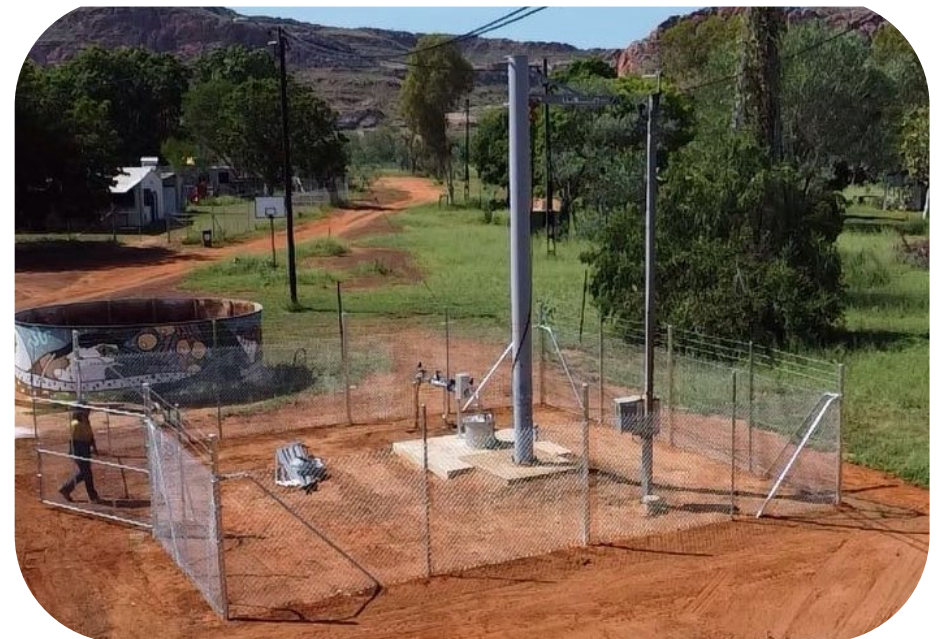
Figure 9: New fencing and bore headworks have reduced the risk of contamination at Jarlmadangah
