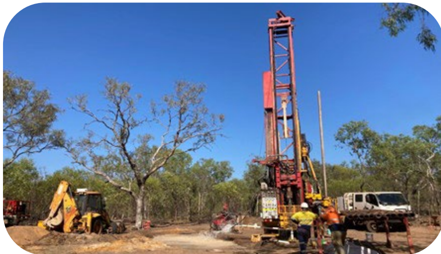
Figure 5: New bores being drilled at Beagle Bay
