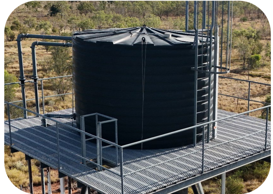
Figure 10: Fitzroy 4 community, Burawa elevated tank
