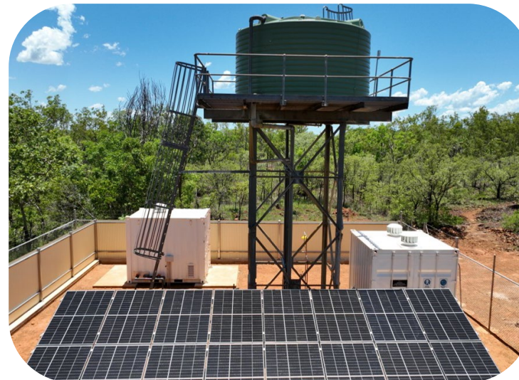
Figure 5: Kandiwal elevated tank and chlorination system
