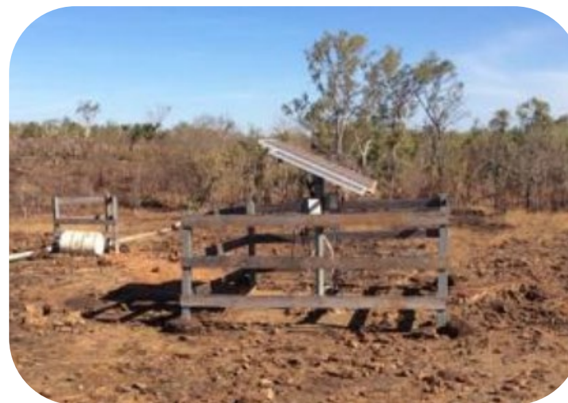
Figure 4: Inadequate fencing around bore
