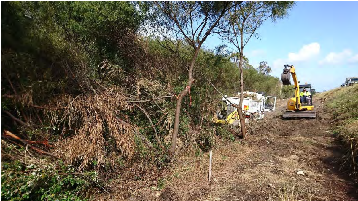
Image 15. Trees with dreys were marked with flagging tape and branches lowered slowly using a small machine to allow BCE personnel to check each drey and move possums if necessary. All material was either carried away, or mulched on site immediately and removed, to avoid creating shelter for animals such as Quenda and Bobtails .
