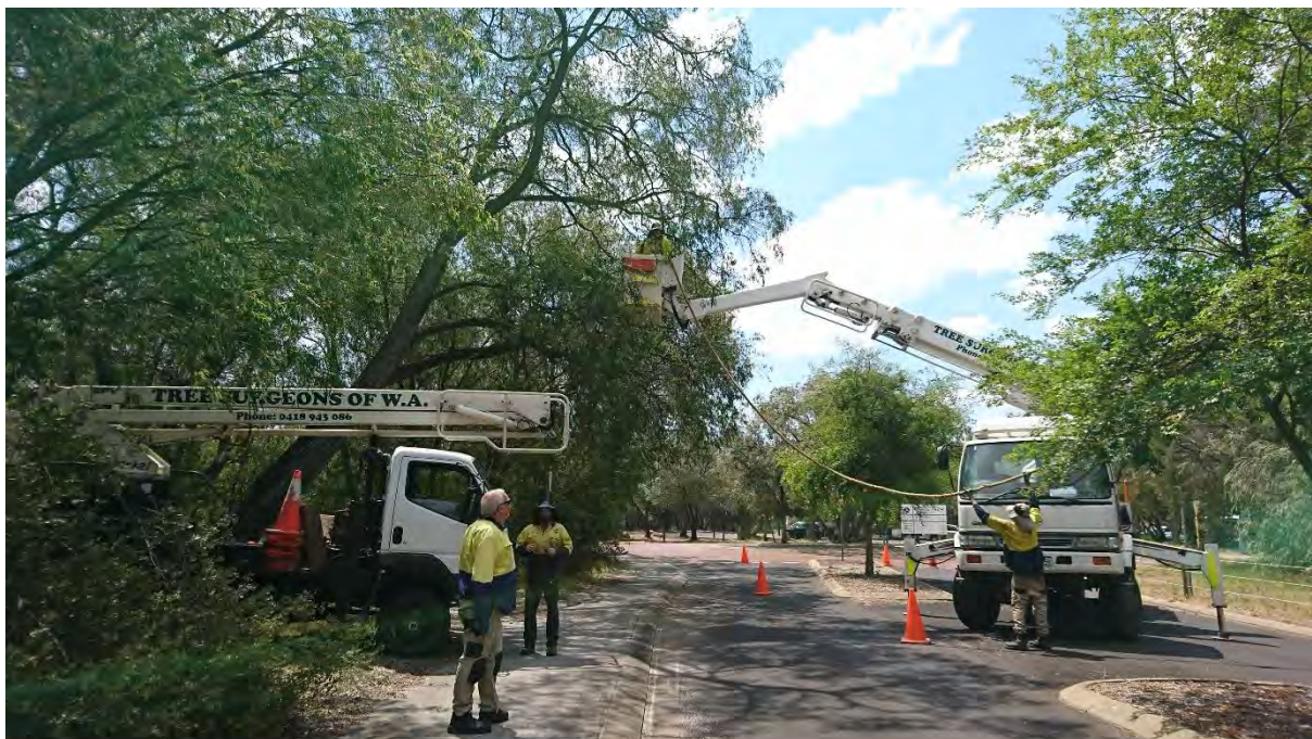
Image 11. Installation of a rope bridge by Tree Surgeons WA at Mary McKillop College, on College Avenue.
