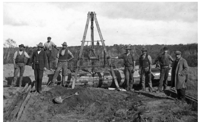
Workers with tripod and winch, lowering pipe near Bandedee. SLWA BA1528/23
