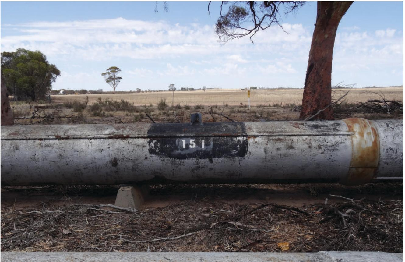
Figure 12. Tammin pipeline section 151km marker detail
