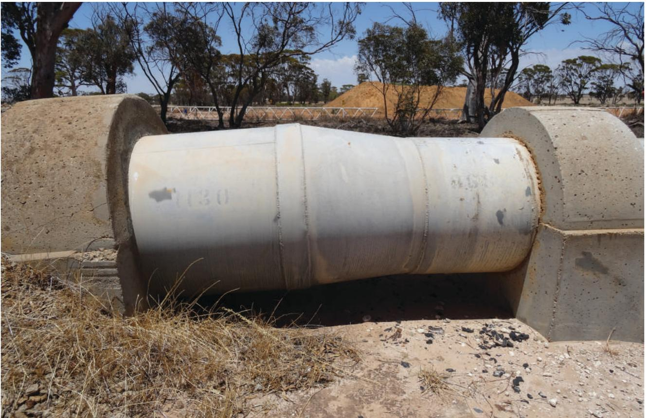
Figure 22. Detail of double concrete bracing arrangement
