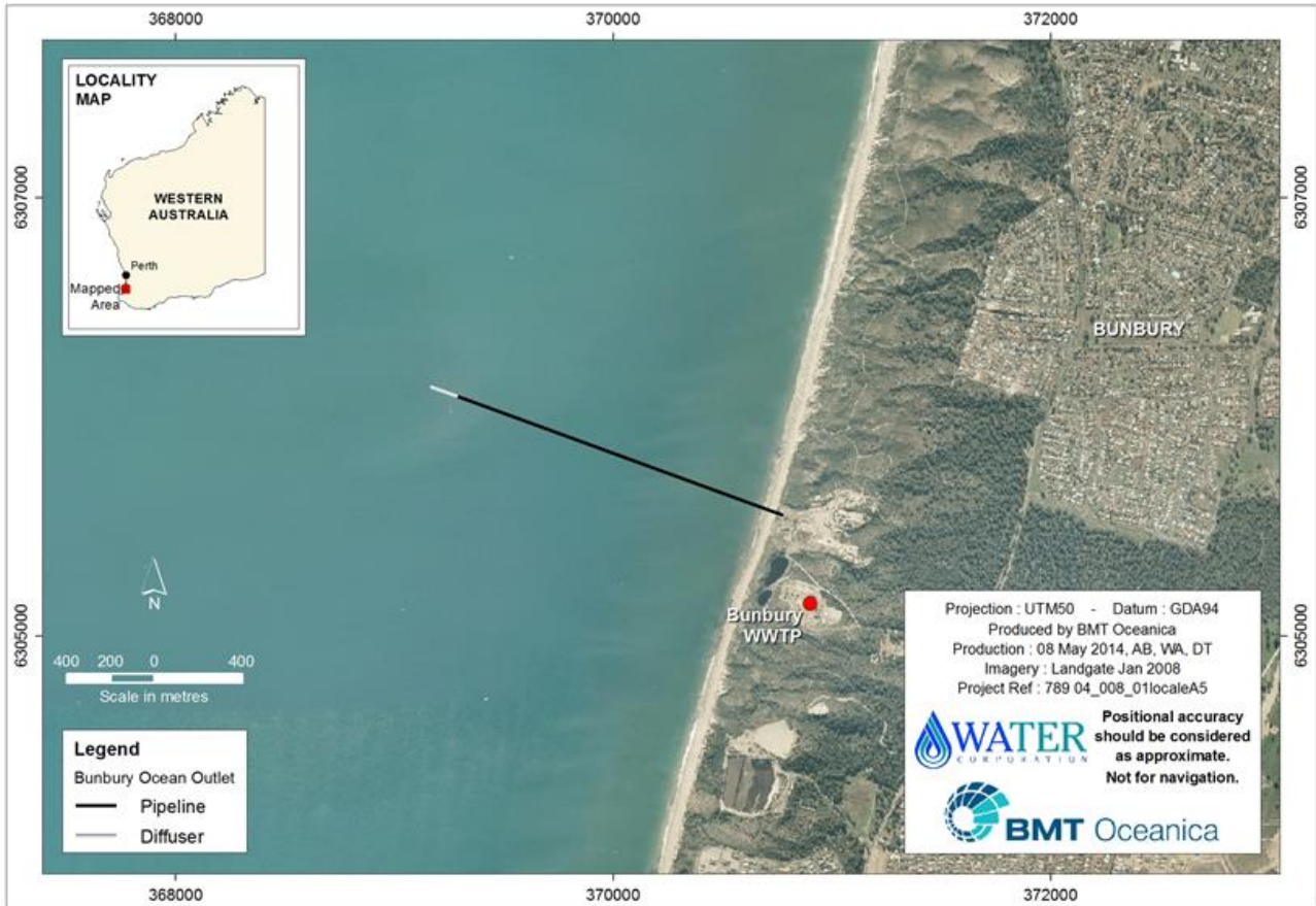
Figure 1.1 Location of the Bunbury Water Resource Recovery Facility and ocean outlet.
