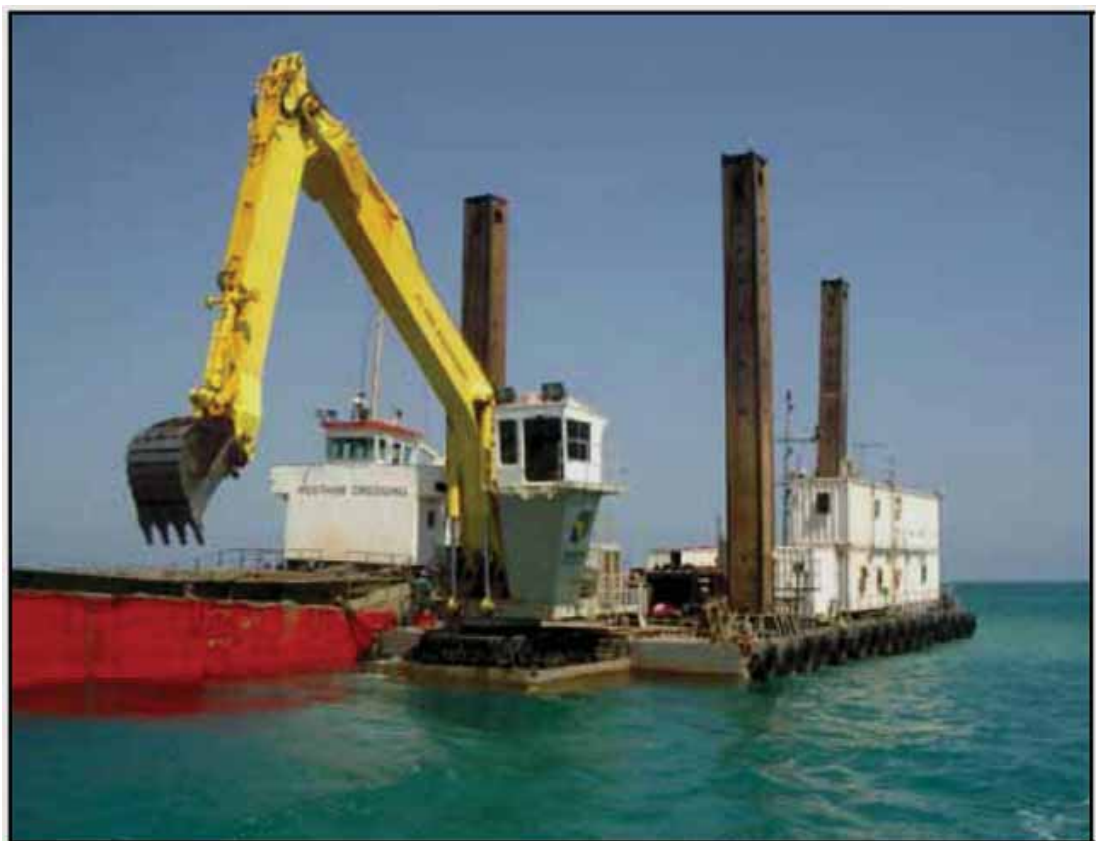
Figure 3-6: Typical backhoe dredge (Atteris 2006)
