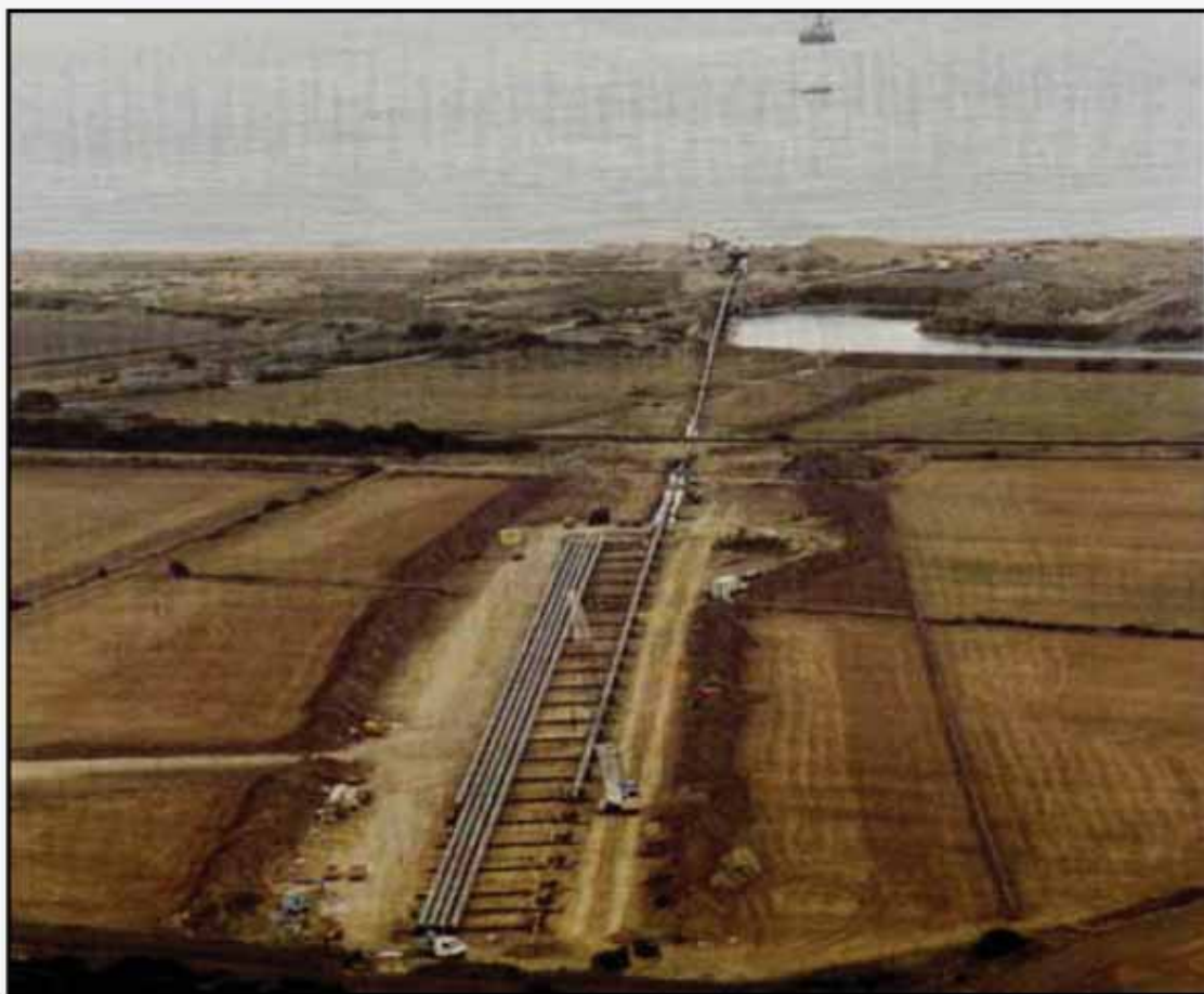
Figure 3-8: A typical pipe sting launch site (Atteris 2006)
