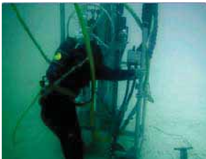
Figure 3-7: Typical diver-operated drill rig
