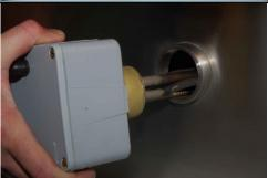
3. Screw the Heater into the Heater Boss on the front side of the unit using Teflon tape to ensure a good seal. **DO NOT CONNECT THE HEATER MUST TO THE ELECTRICAL SUPPLY UNTIL AFTER THE UNIT IS FILLED WITH WATER.**
