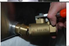
11. Install the self-closing Silt Valve at the inlet end of the unit using the hex fitting provided and Teflon tape. The inlet end may be lifted off the floor to enable this. The handle should be pointing away from the unit to enable it to be opened.
