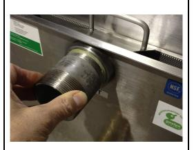
9. The integral vented Flow Control provided with the Goslyn™ should be screwed in the inlet before connecting an inlet line. Its purpose is to regulate the flow so that it does not exceed the capacity of the Goslyn™. Please ensure the narrow end of the cone is closest to the Goslyn™ inlet.
