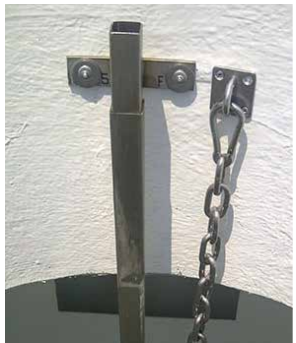
Coalescer Guiderail & Lifting Chain
