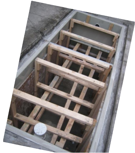
A well braced tank
