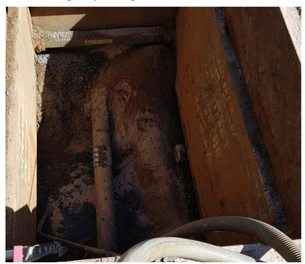
Excavation and repair of an AC pipe in a trench box
