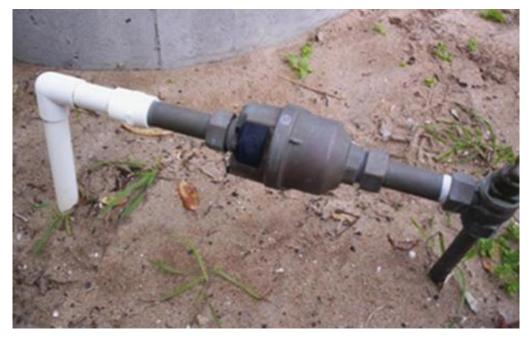
This meter has a plastic vertical pipe and doesn't allow us to fit bridging cables.
