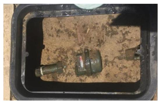
This box is not an approved box and has a build up of soil covering the meter.
