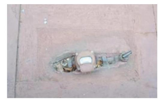
This meter has been covered by concrete and we can't install our sub-meter.
