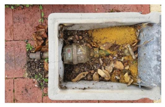
This box is not an approved box and we will not install a sub-meter in this situation.
