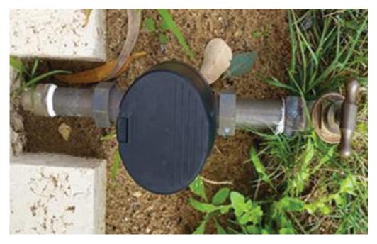
This pipework has been installed in limestone pavers and we will not install our sub-meter.
