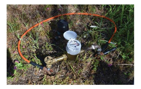
The below photo is an example of the pipework set-up where there is not an existing sub-meter, a piece of poly pipe has been placed where we will install the tails and sub-meter and the unit number is clearly marked.
