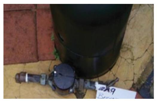
This meter has been positioned too close to a power dome and the pipework is installed in pavers.
