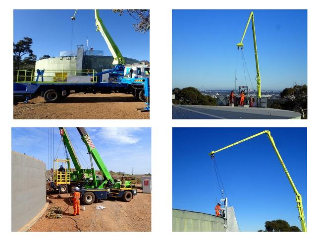
Photo 5 – Use of Sky Hook for safe working on the tank roof.
