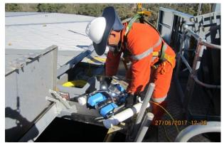
Photo 11 – Tank internal inspection using ROV.
