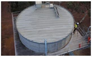
Photo 10 – Inspection of the elevated tank roof using RPA.
