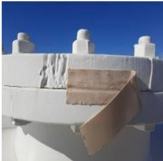
Photo 4. Visco-elastic tape application around a recoated flange is used to prevent under film corrosion and staning.
