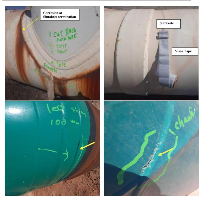
Photo 5. Visco-elastic tape application, where existing Sintakote termination has failed.
