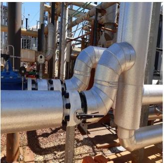
Photo 7. Thermal insulation is installed following completion of Visco-elastic Tape to all pipework and flanges to prevent corrosion under insulation
