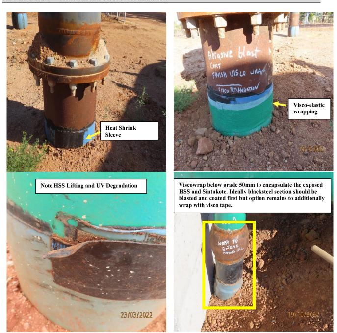
Photo 6. Visco-elastic tape is used on exposed heat shrink sleeve to provide UV protection and to prevent moisture ingress at HSS termination.
