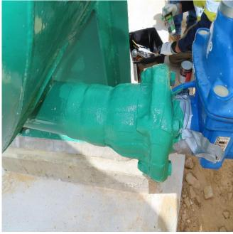
Photo 1. Above ground scour valve offtake before and after visco-elastic tape application.
