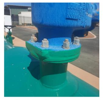
Photo 2. Visco-elastic tape application around coated flange circumference is used to prevent corrosion.
