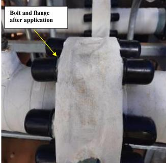
Photo 3. Visco-elastic tape application at the flange gap and bolts to prevent corrosion
