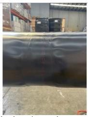
Shrink the sleeve in complete concentric bands starting at the middle of the sleeve and gradually work to the edge of the sleeve.
