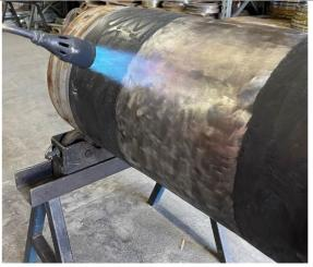
Pre-heat steel to 25°C or 3°C above dew point using the UCC KLON 114KW Gas Torch Kit
