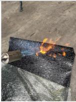
Pre-warm adhesive on sleeve leading edge to ensure good initial bond to steel and Sintakote.
