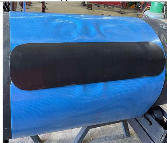
Place the closure patch centrally on the sleeve overlap and pat down firmly.
