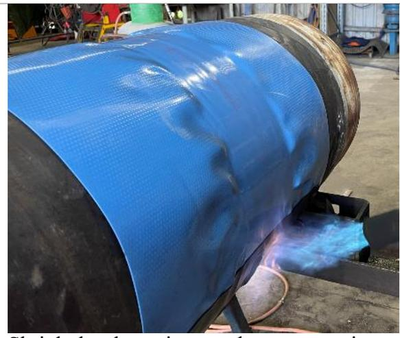
Shrink the sleeve in complete concentric bands starting at the middle of the sleeve and gradually work to the edge of the sleeve.
