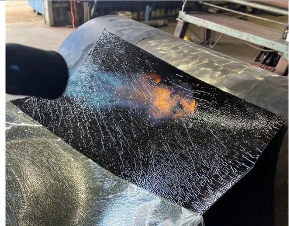
Pre-warm adhesive on sleeve leading edge to ensure good initial bond to steel and Sintakote.
