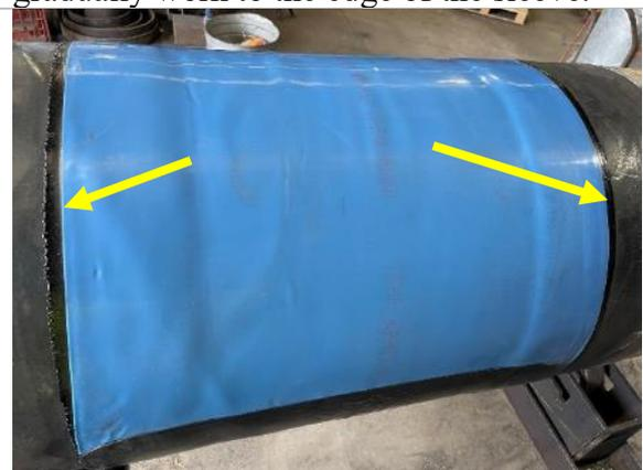
Finished sleeve with adhesive oozing.
