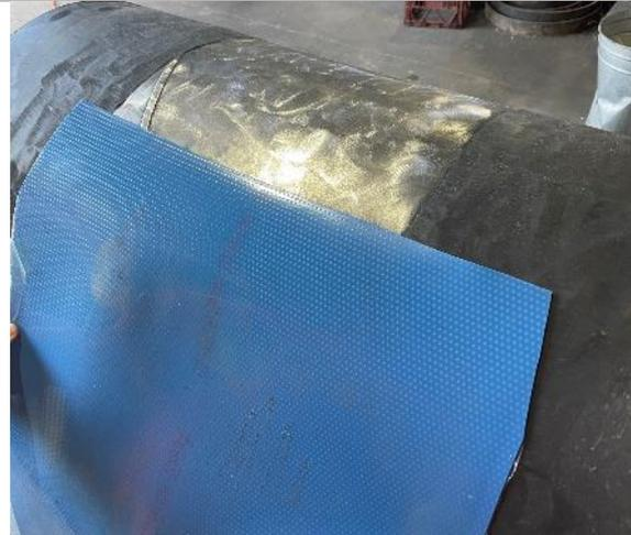
Chamfer leading edge of sleeve 25mm x 50mm lead in approx.
