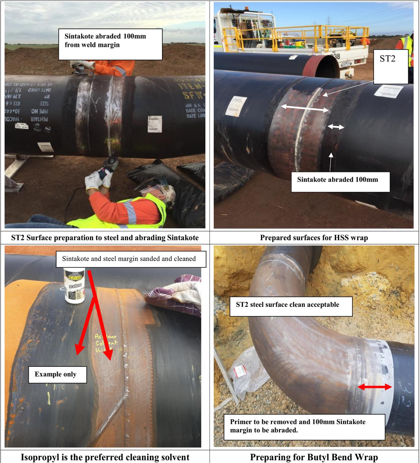
Figure 5: Sintakote & Steel Surface Preparation
