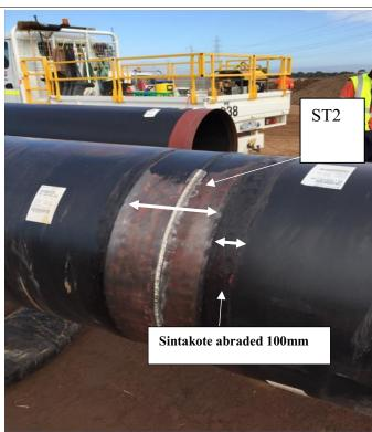
ST2 Surface preparation to steel and abrading Sintakote
