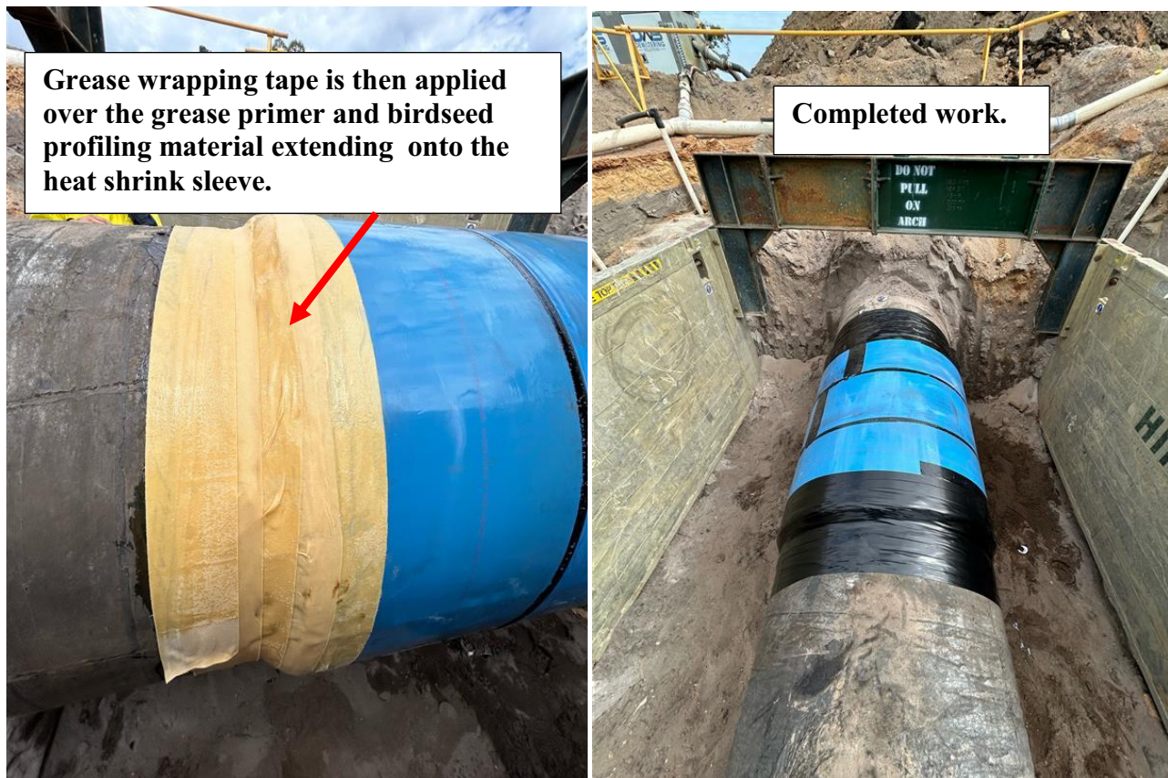
Figure 4: Petrolatum system over old CTE/bituminous lining to HSS
