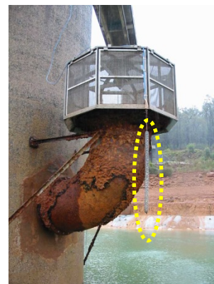
Photo 6 – Sacrificial Anode inspection on the intake tower.
