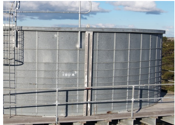
Photo 13 - Tank external wall and handrails.
