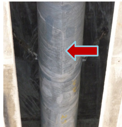
Photo 4 – Pipeline under the bridge.
