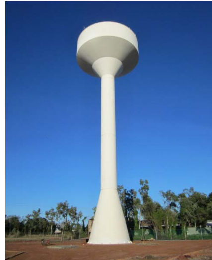
Photo 2 – Elevated steel tank.
