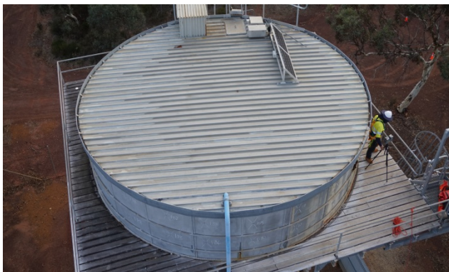
Photo 10 –Elevated tank roof and platform.
