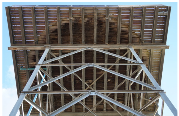
Photo 11 – Underside of tank platform.
