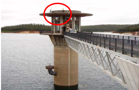
Photo 5 – Inspection of Intake tower in the Dam by conventional inspection approach.
