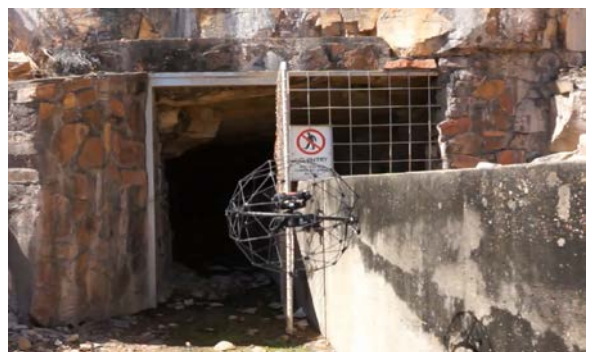
Photo 19 - Inspection of a tunnel using a caged RPA
