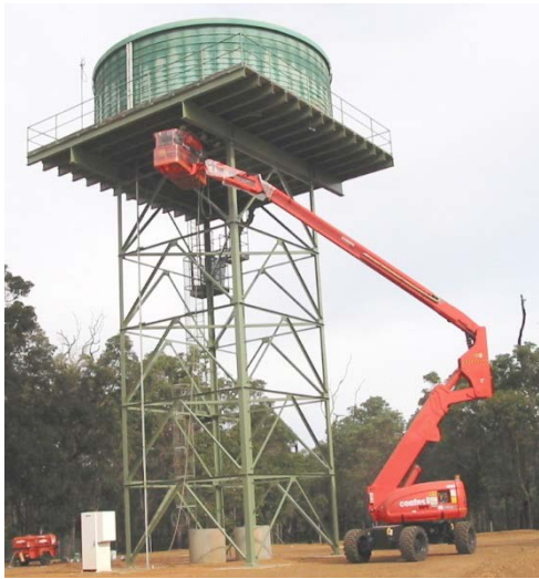
Photo 1 – Elevated steel tank.
