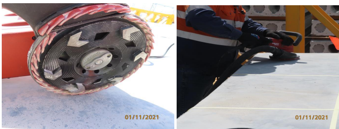
Figure 1 Typical surface preparation by grinding
