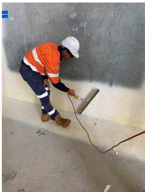
Figure 8 Example of spark test
