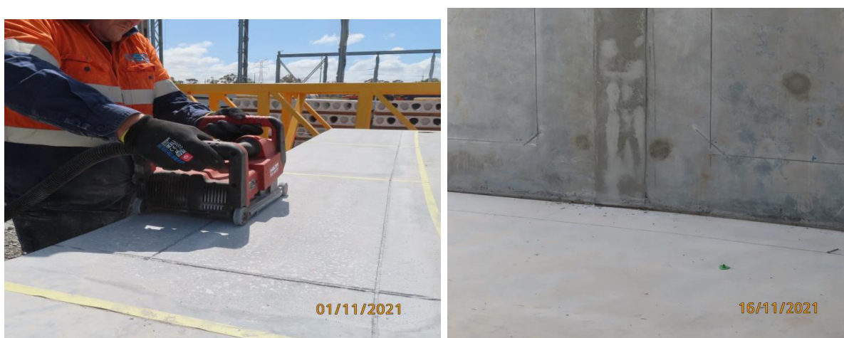
Figure 2 Typical termination groove
