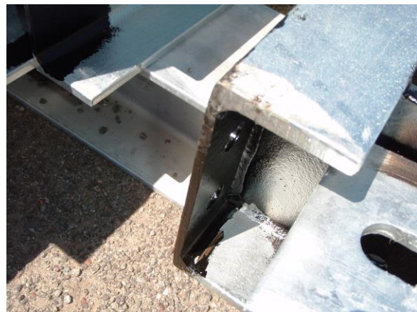
Photo 3 - Coating on the galvanised beam to prevent crevice/dissimilar metal corrosion.
