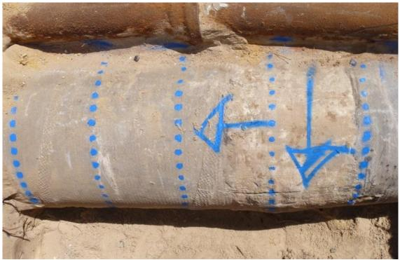
*Figure 4 – DN610 MSCL pipe with factory-applied asbestos cement wrap coating (left of image) and field-applied asbestos mortar over the joint (right).*
