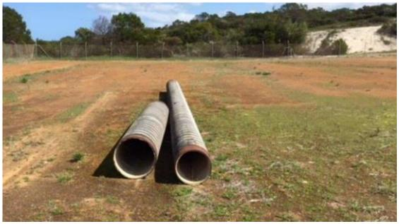
Figure 25 - Weathered asbestos coal tar coated pipe at Thompson Street WPS, Esperance. Note the spiral wrap, remnant whitewash and coating colour weathered to light grey.
