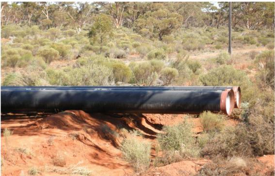
Figure 32 - New Sintakote pipe prior to installation. Note the smooth seamless black coating.
