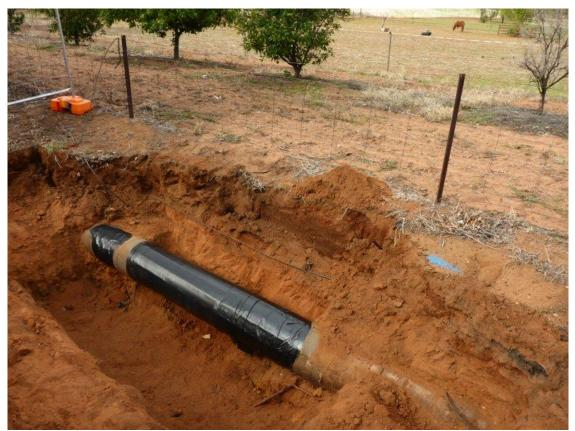
*Figure 16 - DN300 Damaged asbestos coal tar coating repaired using non-hazardous repair system (primer, butyl mastic strip and PVC tape)*.
