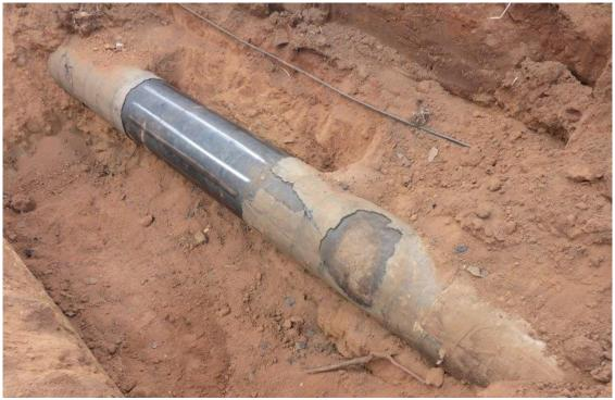
Figure 15 - DN300 Damaged asbestos coal tar coated pipe at York.
