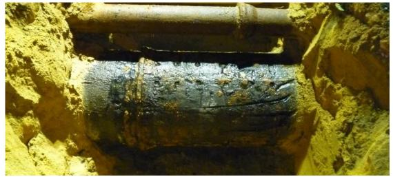
Figure 2 - DN760 pipe with bitumen coating without wrapping fabric installed in Nedlands in 1934.
