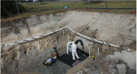
*Figure 17 – Removal of asbestos coal tar coating from DN1400 main prior to welding in East Rockingham. Note the spiral wrapping of the bandage and intact whitewash coating.*
