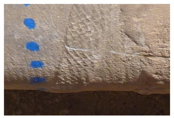
*Figure 5 - A closer look of the coarse weave of the asbestos bandage is evident at the overlap; hand-applied asbestos mortar over the field joint is at the right of the image.*
