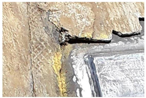
Figure 9 - - DN 1065 Canning Trunk Main, Albany Hwy, Maddington. Close-up of asbestos cement bandage
