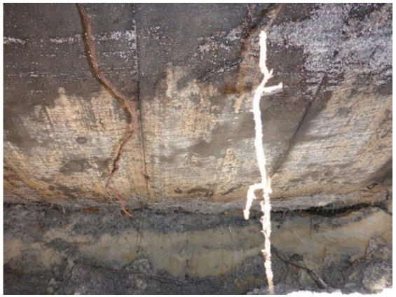
*Figure 19 – Underside of the DN1220 Serpentine trunk main, Riverton (installed 1953). Note the remnant whitewash coating.*
