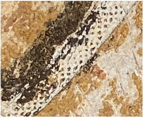
Figure 7 - DN1065 Canning Trunk Main, Albany Hwy, Maddington. Close-up of bandage overlap.
