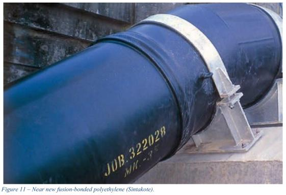
*Figure 11 – Near new fusion-bonded polyethylene (Sintakote).*
