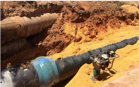
Figure 34 - New Sintakote pipe (foreground) during installation. Note the smooth seamless black surface and the spiral pipe weld seam evident through the coating. Older Asbestos CTE coated pipe in the background.
