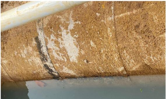
*Figure 6 – DN1065 Canning Trunk Main, Albany Hwy, Maddington. Note the coarse weave of the asbestos bandage evident at the overlap of the wrap.*
