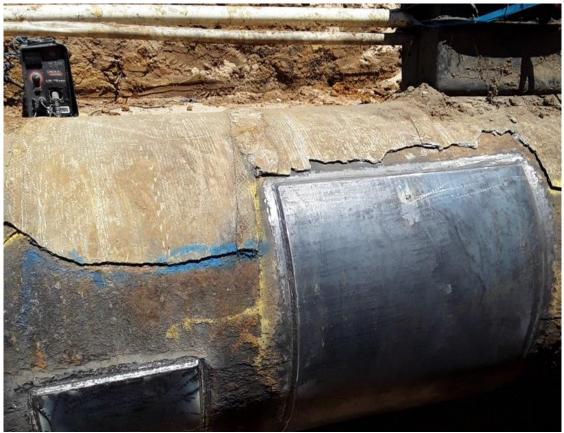
*Figure 8 – DN 1065 Canning Trunk Main, Albany Hwy, Maddington. Asbestos cement bandage removed for pipe repair.*
