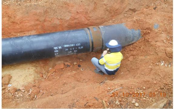
*Figure 33 - New Sintakote pipe during installation. Note the smooth seamless black surface and the evident spiral pipe weld seam under the coating.*
