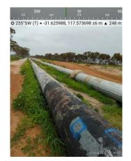
Figure 1 – Decommissioned DN760 locking bar pipe installed above ground near Tammin. This pipe was originally buried but was reinstalled above ground in the 1930s. This example includes various coatings including remnants of the original hot-dipped bitumen coating.
