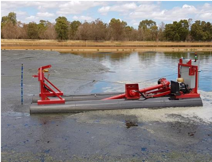
Figure 6-2: Online unmanned dredge
