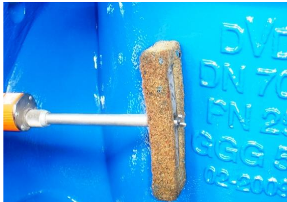
Figure 5: Low Voltage Test Continuity Test using Wet Sponge method
