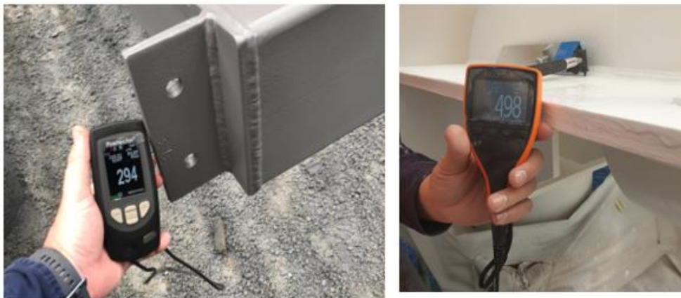
Figure 4: Measurement of DFT using electronic gauge.
