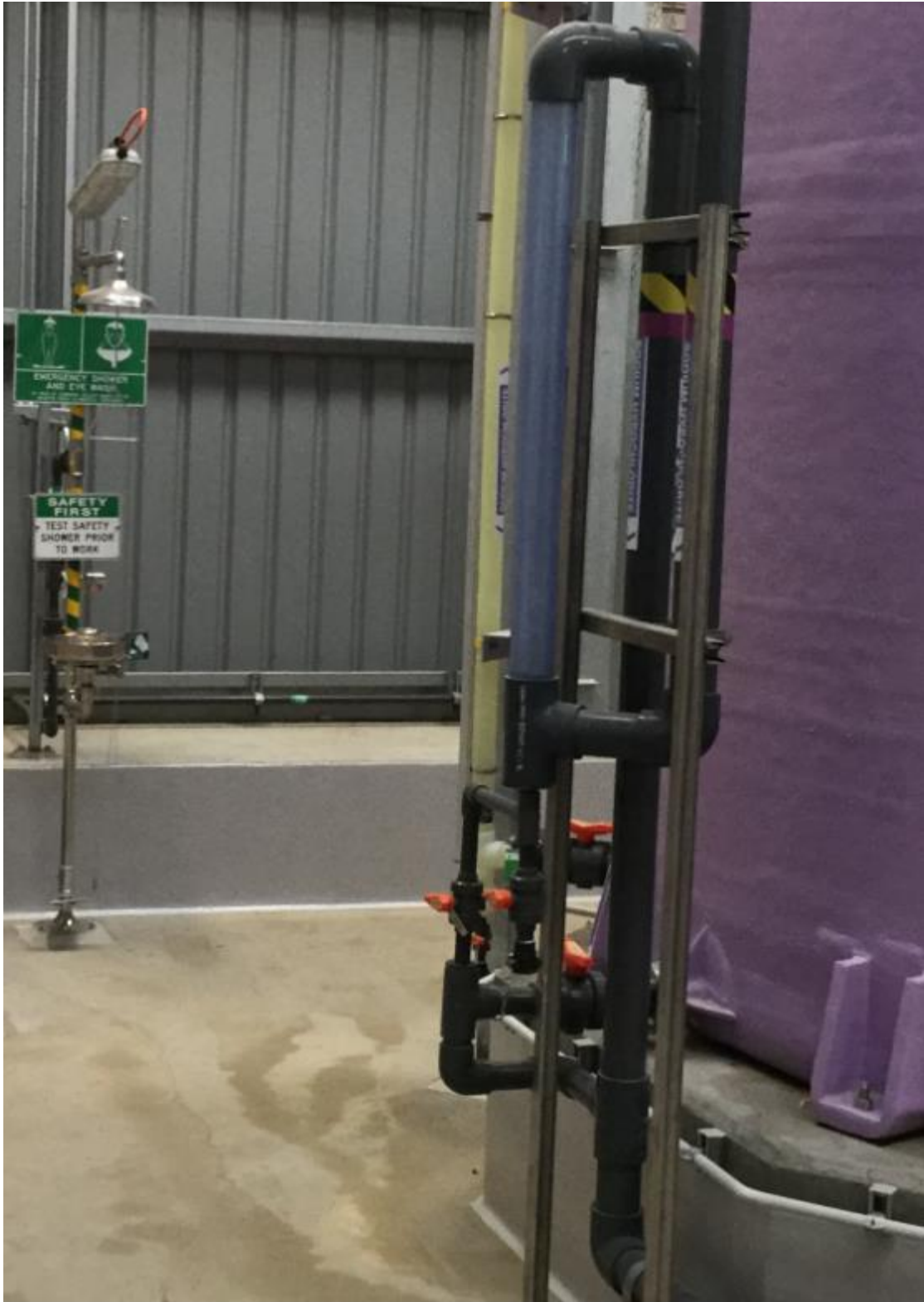
Figure 5-1: Overflow line with a transparent fillable seal pot visible from load-in panel
