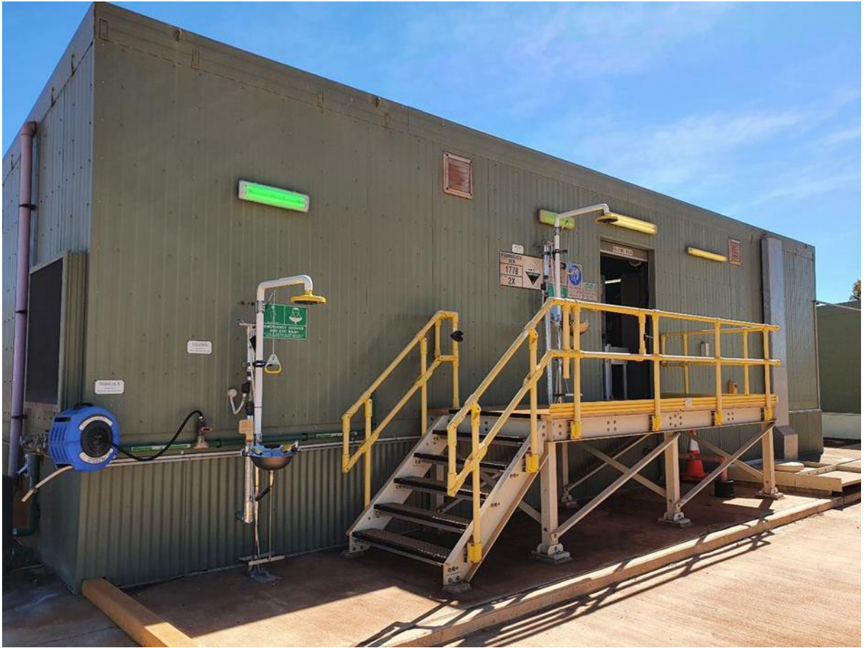
Figure 5-1: Continuation of raised platform outside roller door
