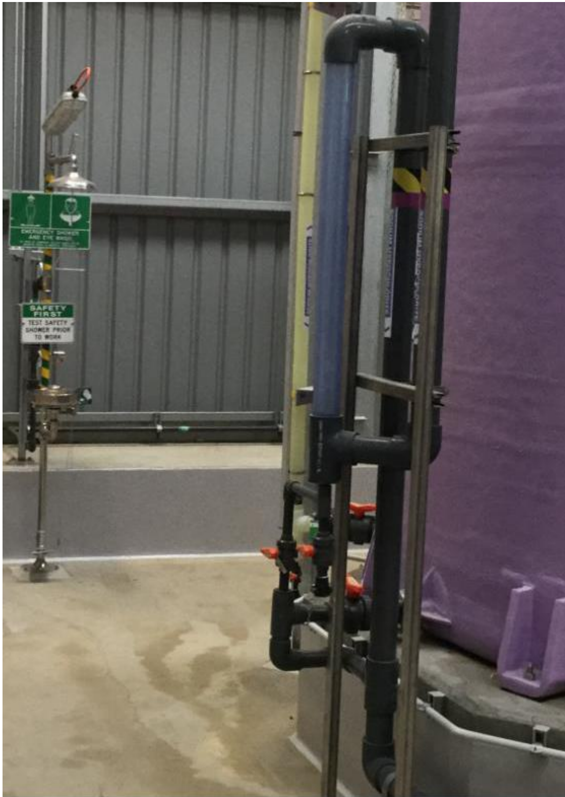
Figure 5-2: Overflow line with a transparent fillable seal pot visible from load-in panel
