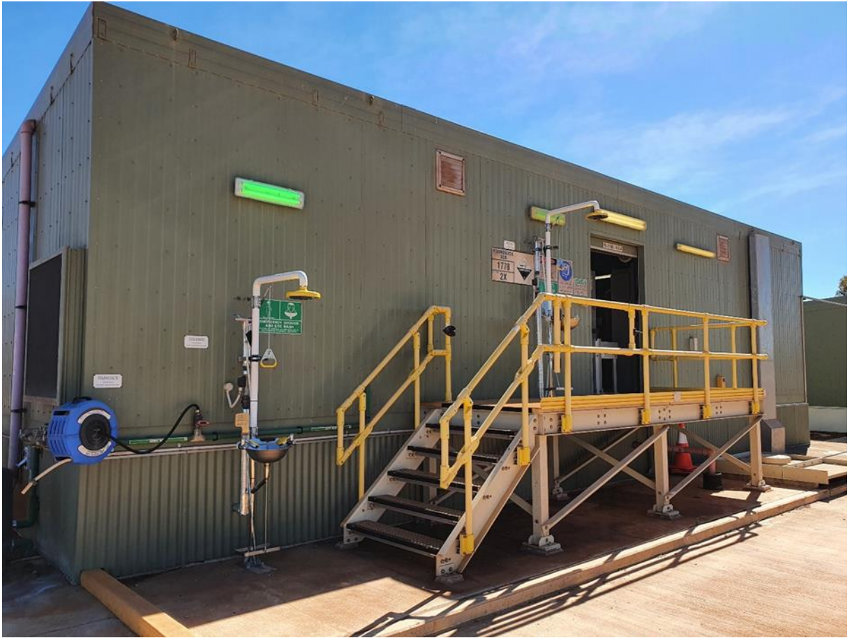
Figure 5-1: Continuation of raised platform outside roller door
