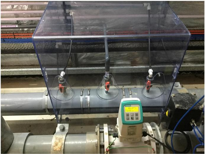
Figure 7-3: Local dose point enclosure: covers the pipework and fittings at the dose point. Tear-drops allow access for valve operation
