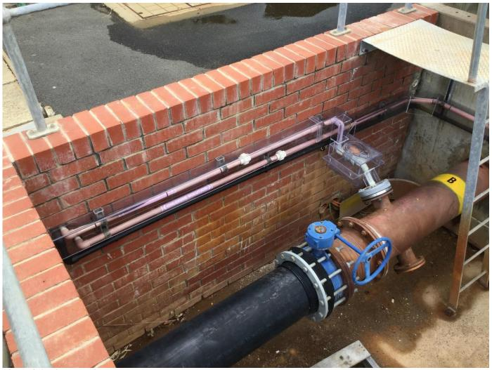
Figure 8-1: Pipe cover is segmented
