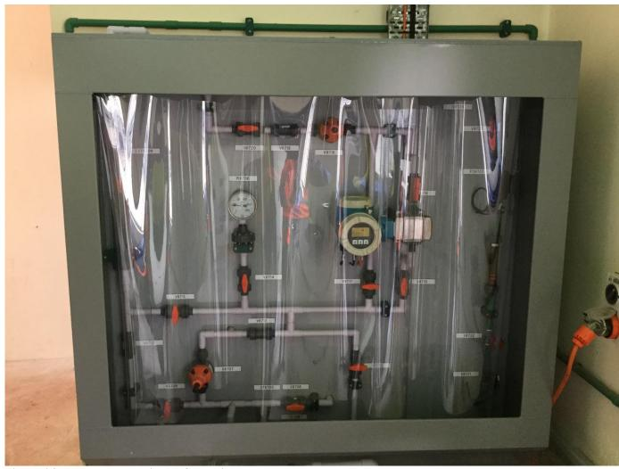
Figure 6-2: Low enclosure with PVC curtains
