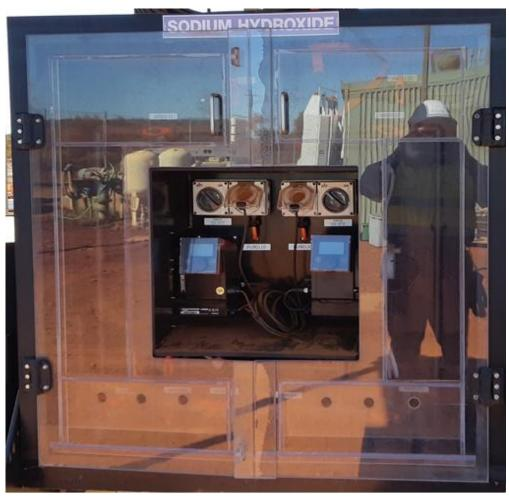
Figure 5-1: Medium Enclosure with cutout for pump and electrical connections
