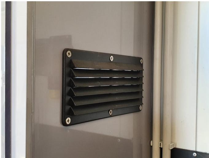
Figure 5-4: Side mounted enclosure vent, angled to prevent direct spray of chemical out
