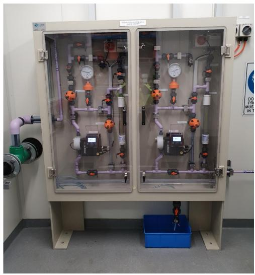
Figure 5-2: Medium Enclosure – doesn't include pump and electrical cutouts but cable duct is provided and electrical connections are mounted high (low corrosivity chemical application)
