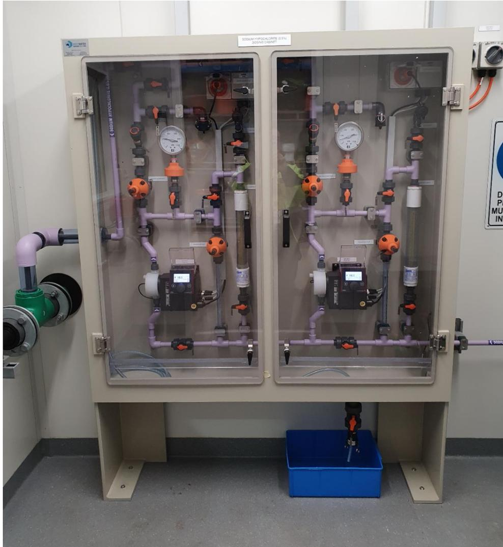
**Figure 5-2: Medium Enclosure – doesn't include pump and electrical cutouts but cable duct is provided and electrical connections are mounted high (low corrosivity chemical application)**
