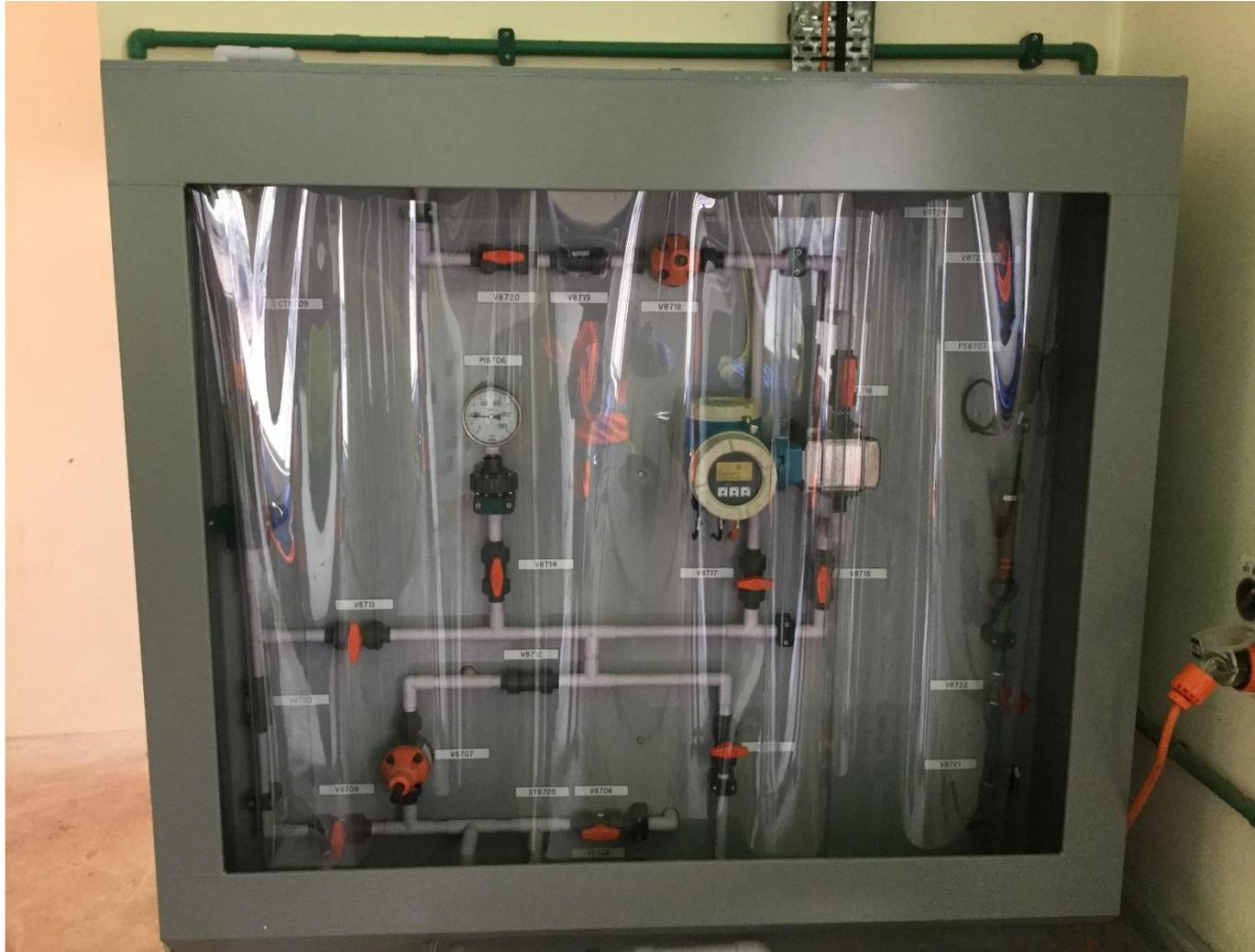
Figure 6-2: Low enclosure with PVC curtains
