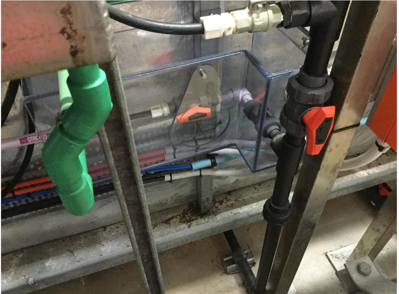
**Figure 7-4: Local dose point enclosure: covers the pipework and fittings at the dose point despite a change in direction. Tear-drop allows access to main isolation valve**
