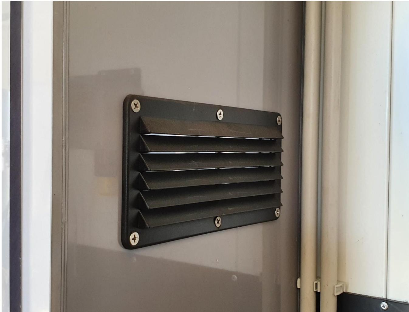
**Figure 5-4: Side mounted enclosure vent, angled to prevent direct spray of chemical out**
