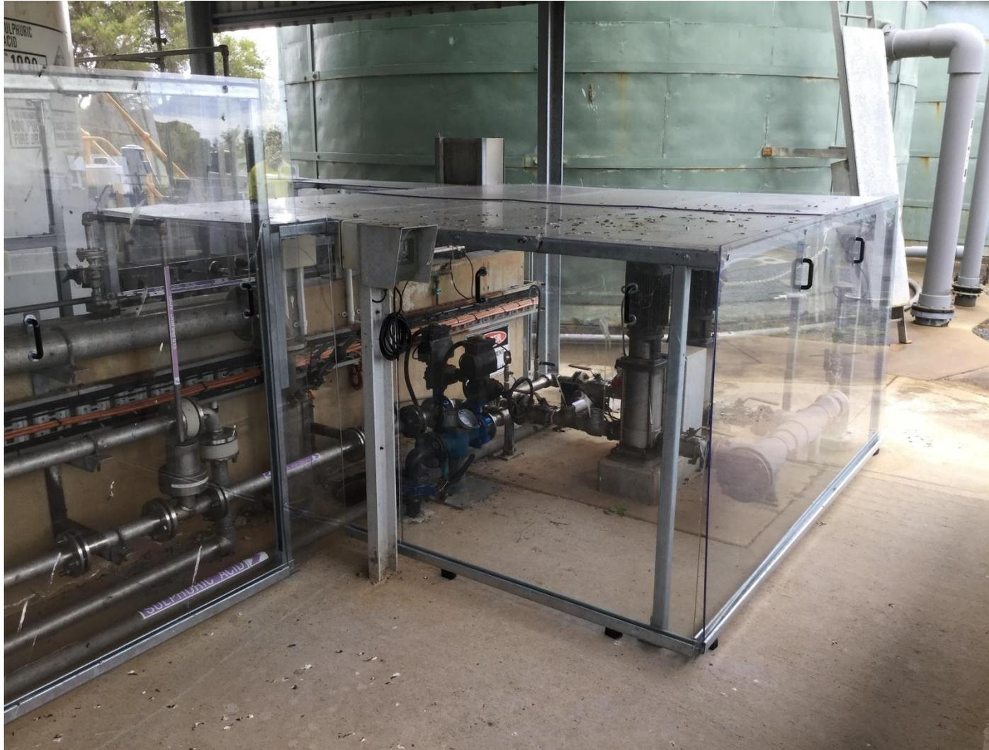
**Figure 5-5: Enclosure retrofit – enclosure will prevent spray from impacting personnel (acid will spread across concrete flooring, but, this presents a lower hazard level)**
