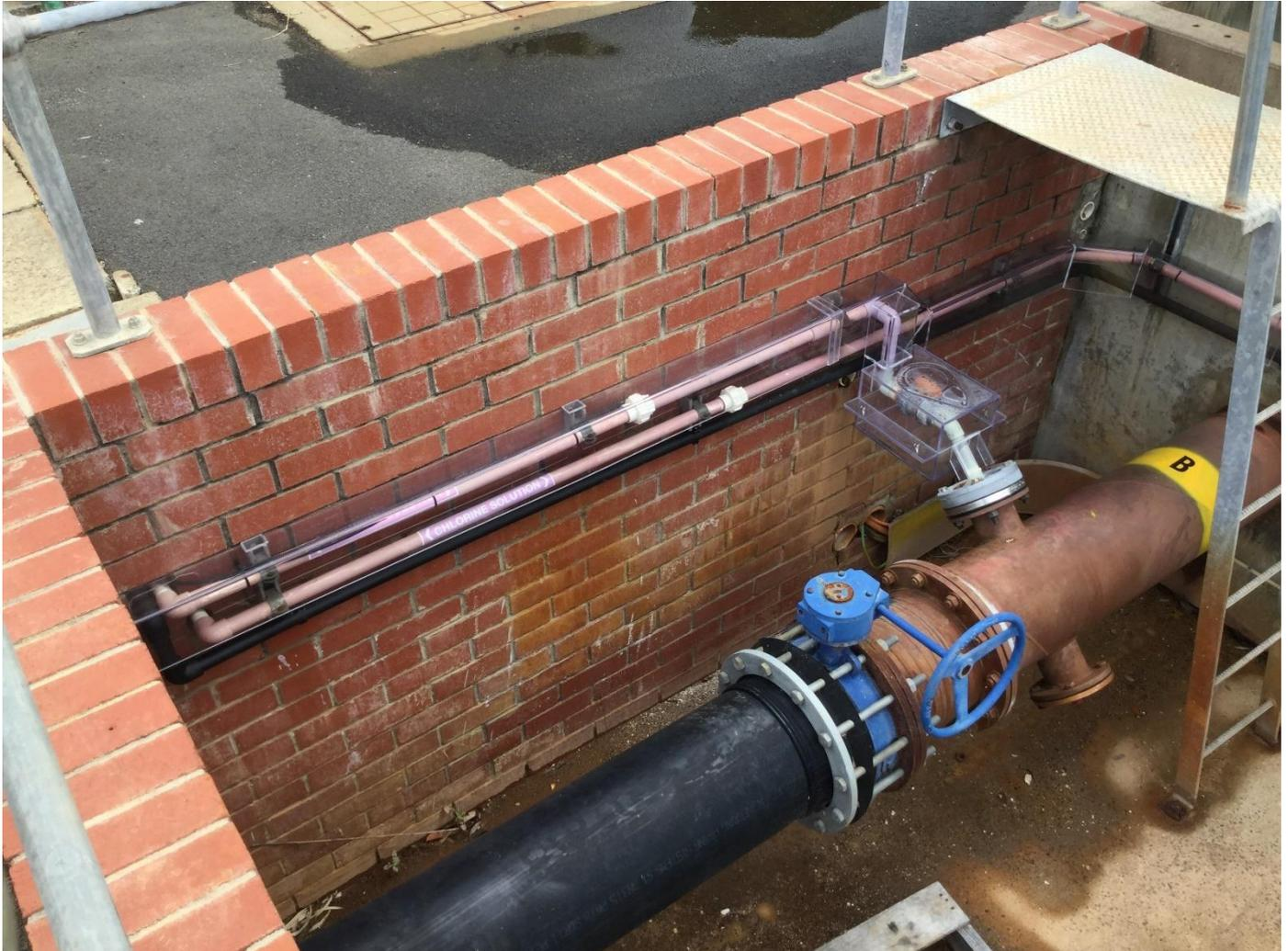
**Figure 8-1: Pipe cover is segmented**
