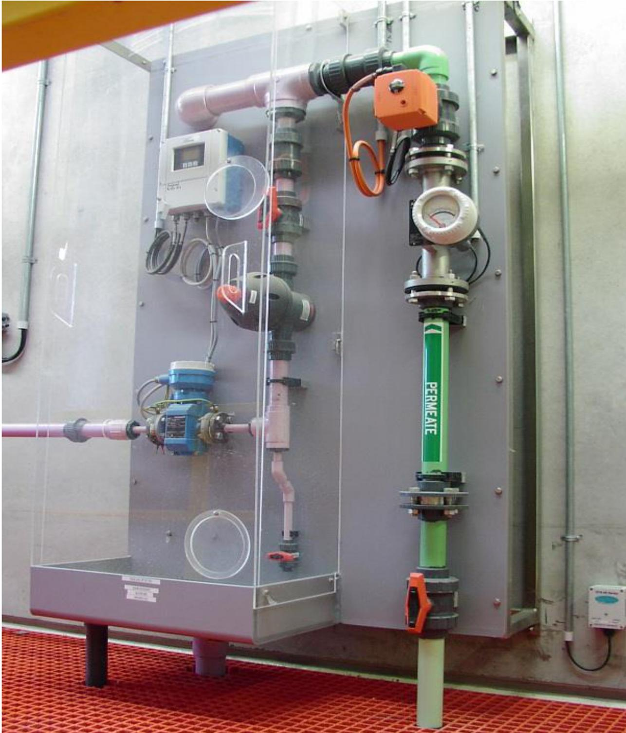
**Figure 7-2: Dose Point: Hatches provided allow operator access to frequently operated valves without having to remove perspex box**
