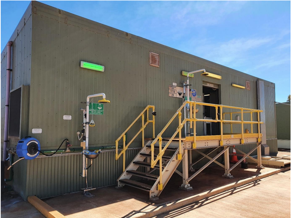
Figure 4-1: Example of a raised load-in platform
