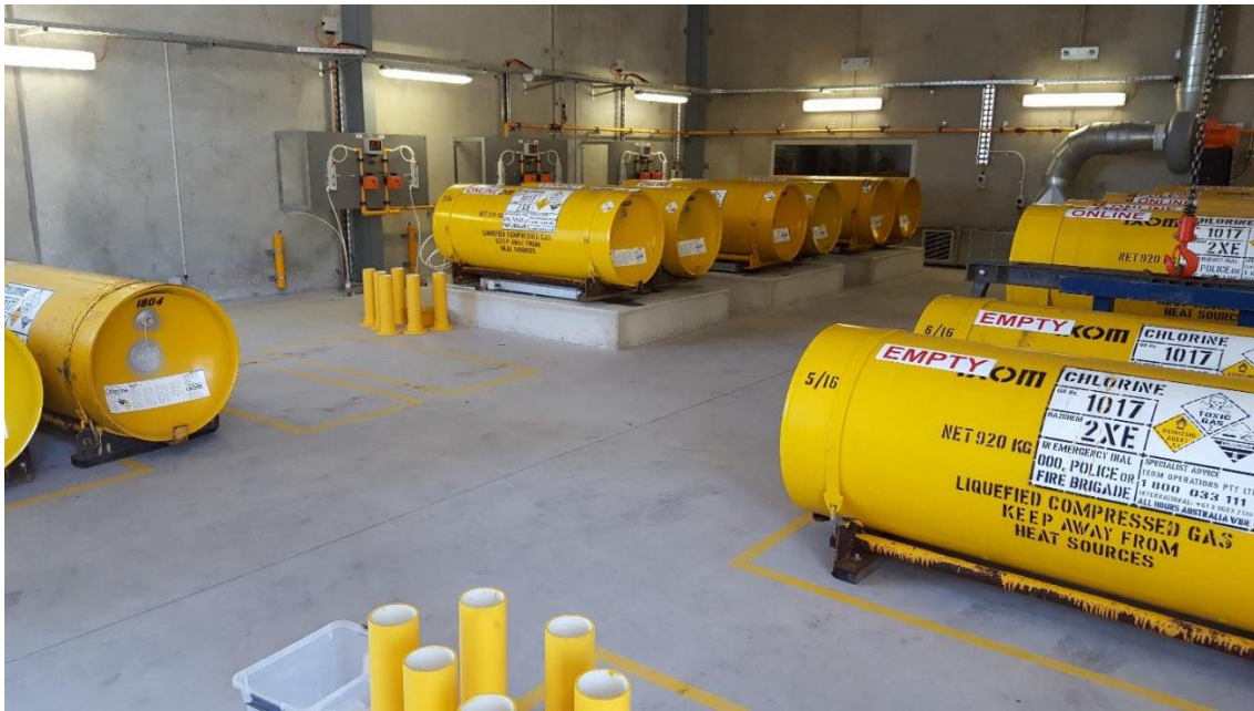
Figure 5: Full view of chlorine containment room (taken from the truck drive through bay)
