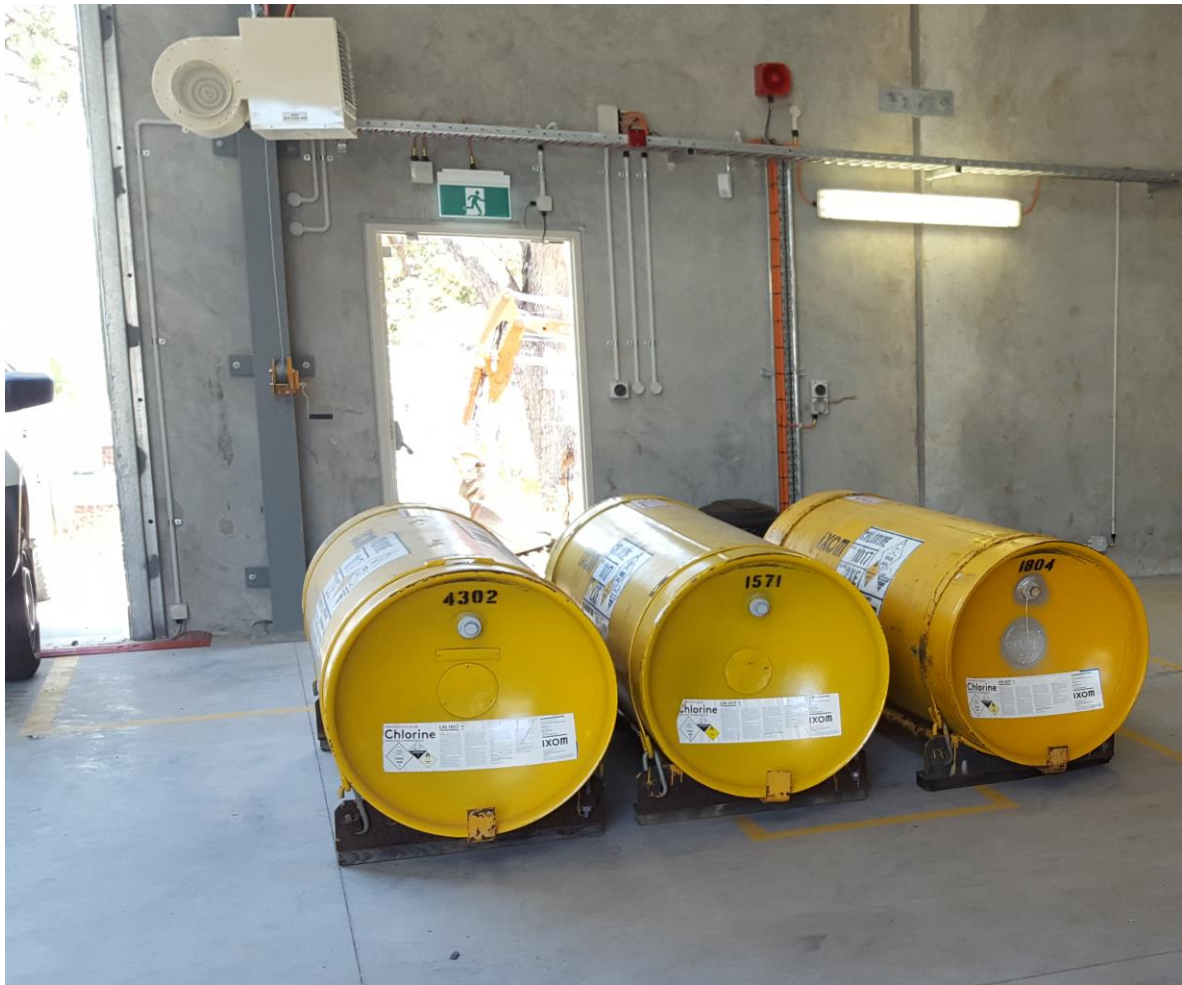
Figure 2: View of emergency exit door
