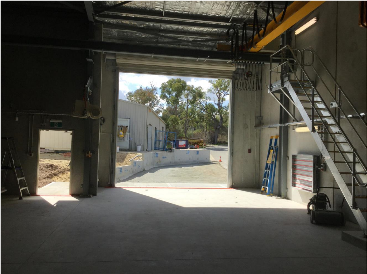
Figure 4: Truck drive-in facility roller door and gantry crane access
