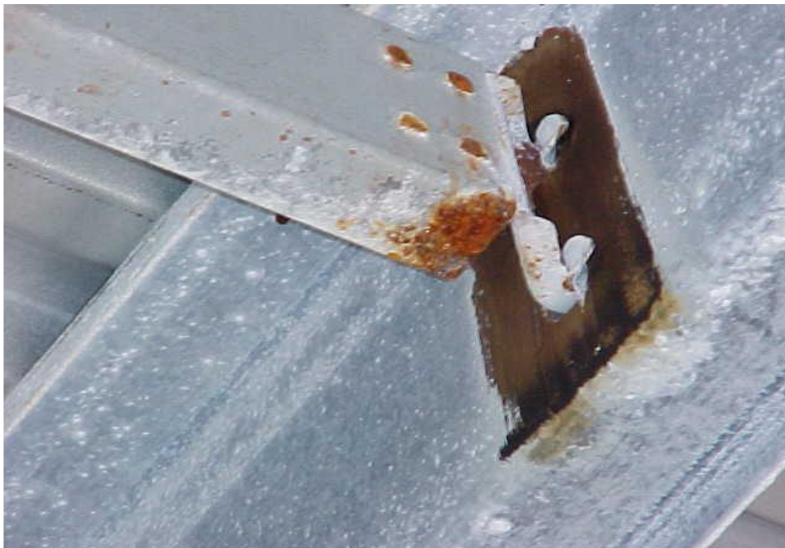
1. Corrosion of Universal Beam at Chlorine Dosing Point
