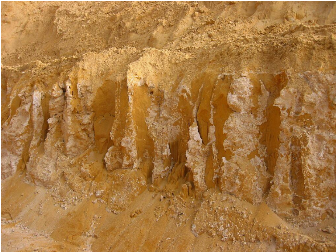
2002 Tamworth Hill Reservoir Solution Pipes in Weak Honeycomb Limestone Foundation
