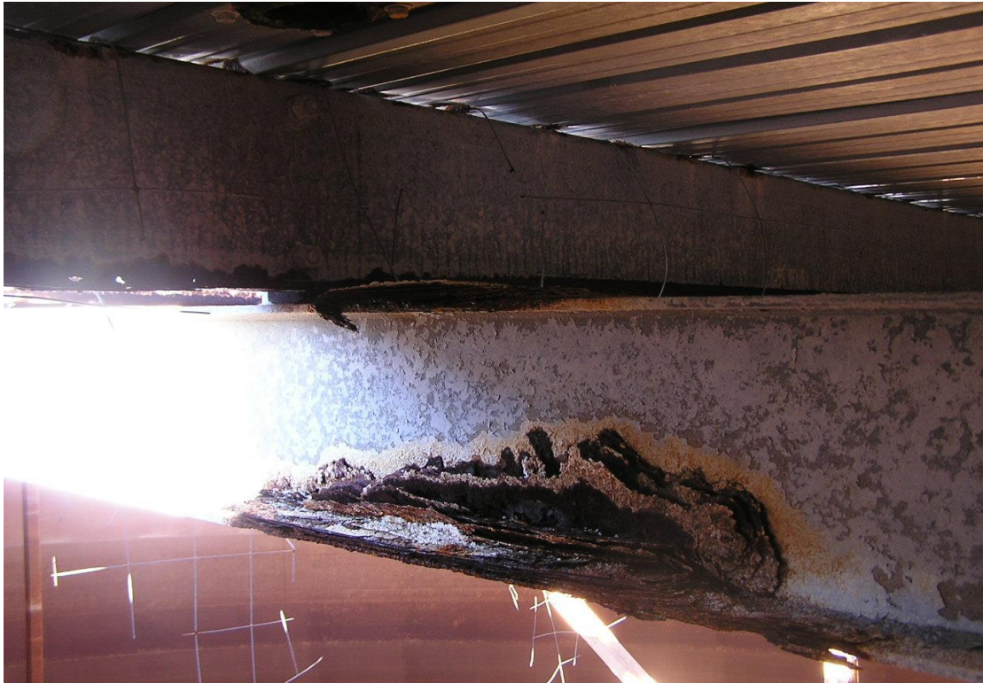
1. Corrosion of Universal Beam at Chlorine Dosing Point
