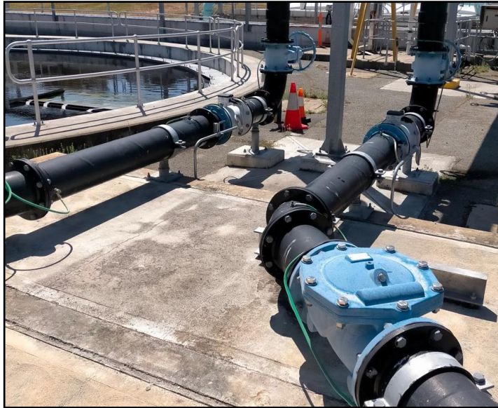
Figure 17: Magflow meters on RAS pipework at Subiaco WRRF
