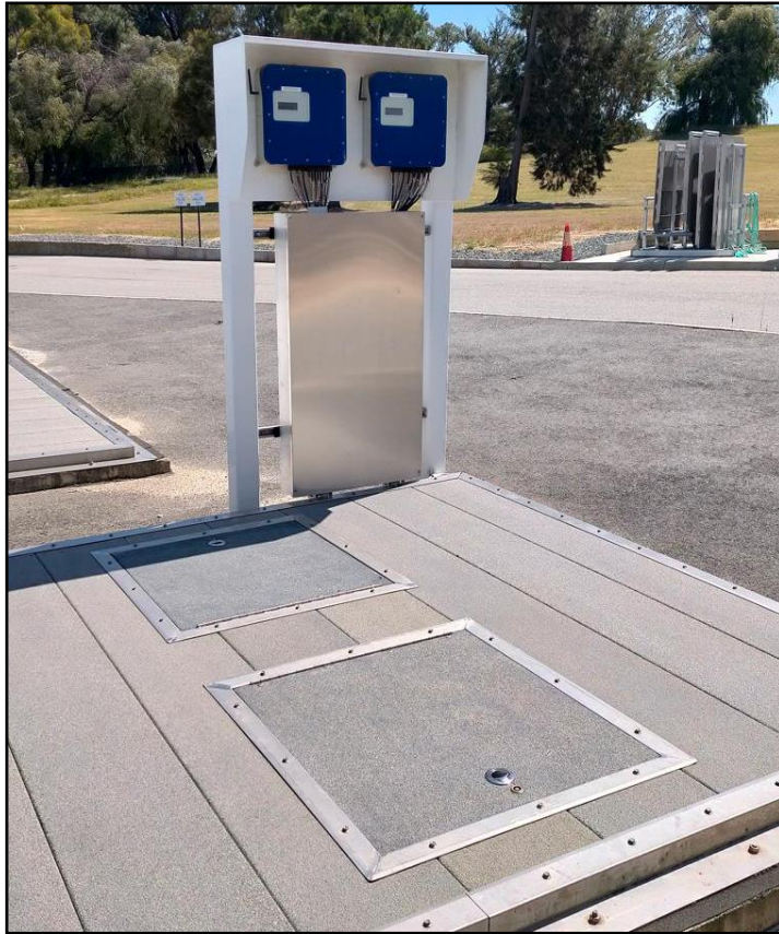
Figure 30: Transient time flow meter installed to measure inflow at the Subiaco WRRF
