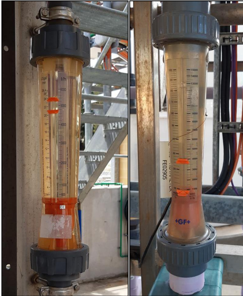
Figure 23: Various rotameters, left – 6,000L/hr, right – 15,000L/hr
