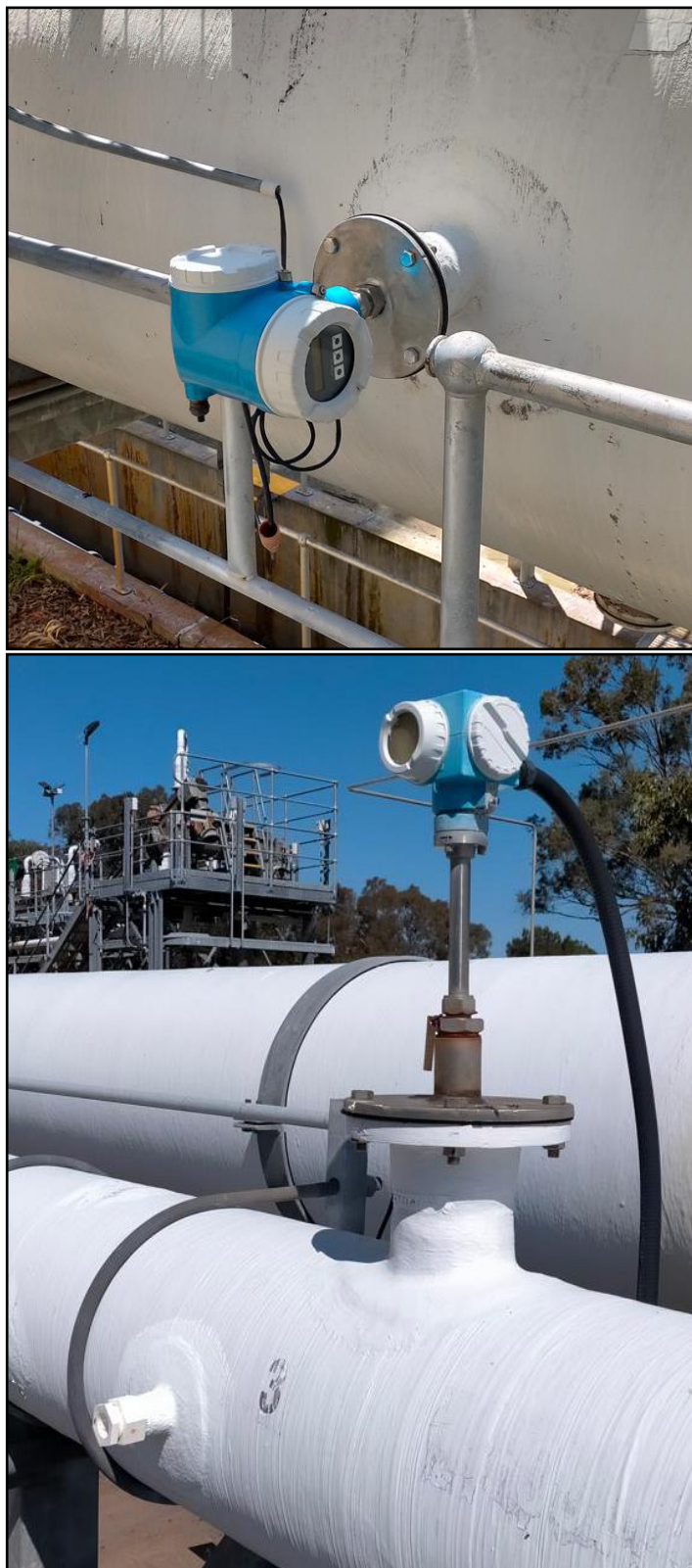
Figure 32: Thermal mass flow meters installed on odour collection pipework.
