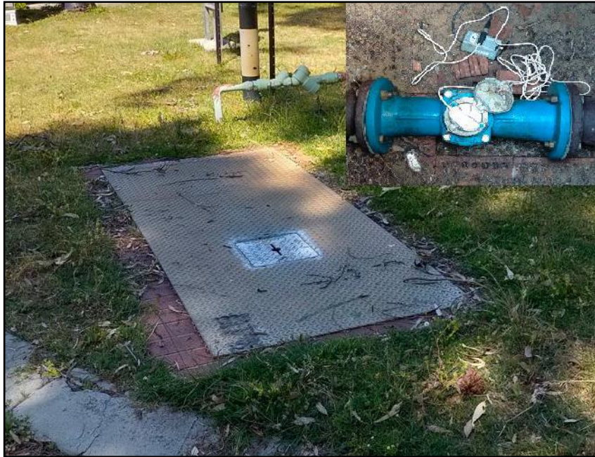
Figure 21: Mechanical flow meter with smart meter add-on. Installed in a below ground pit.
