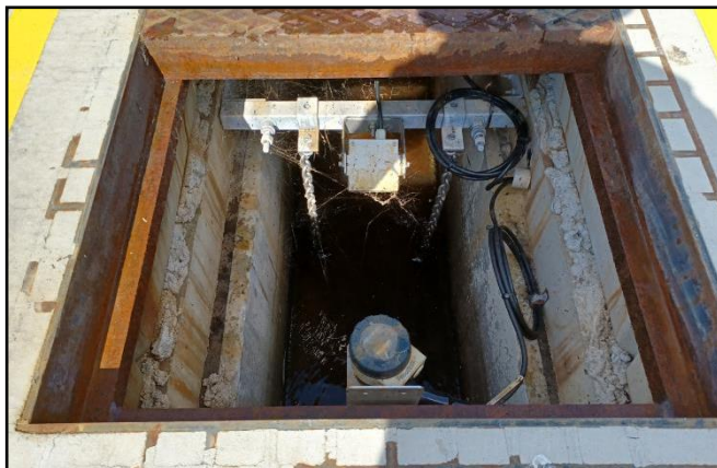
Figure 31: Radar flow meter (velocity and level instruments) installed on the outlet of each of the SST's at Subiaco WRRF.
