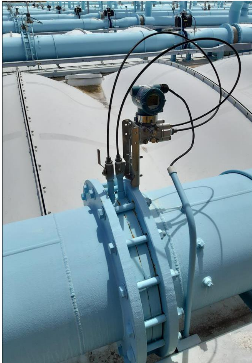
Figure 35: An Orifice plate flowmeter installed on the blower aeration pipework at Subiaco WRRF
