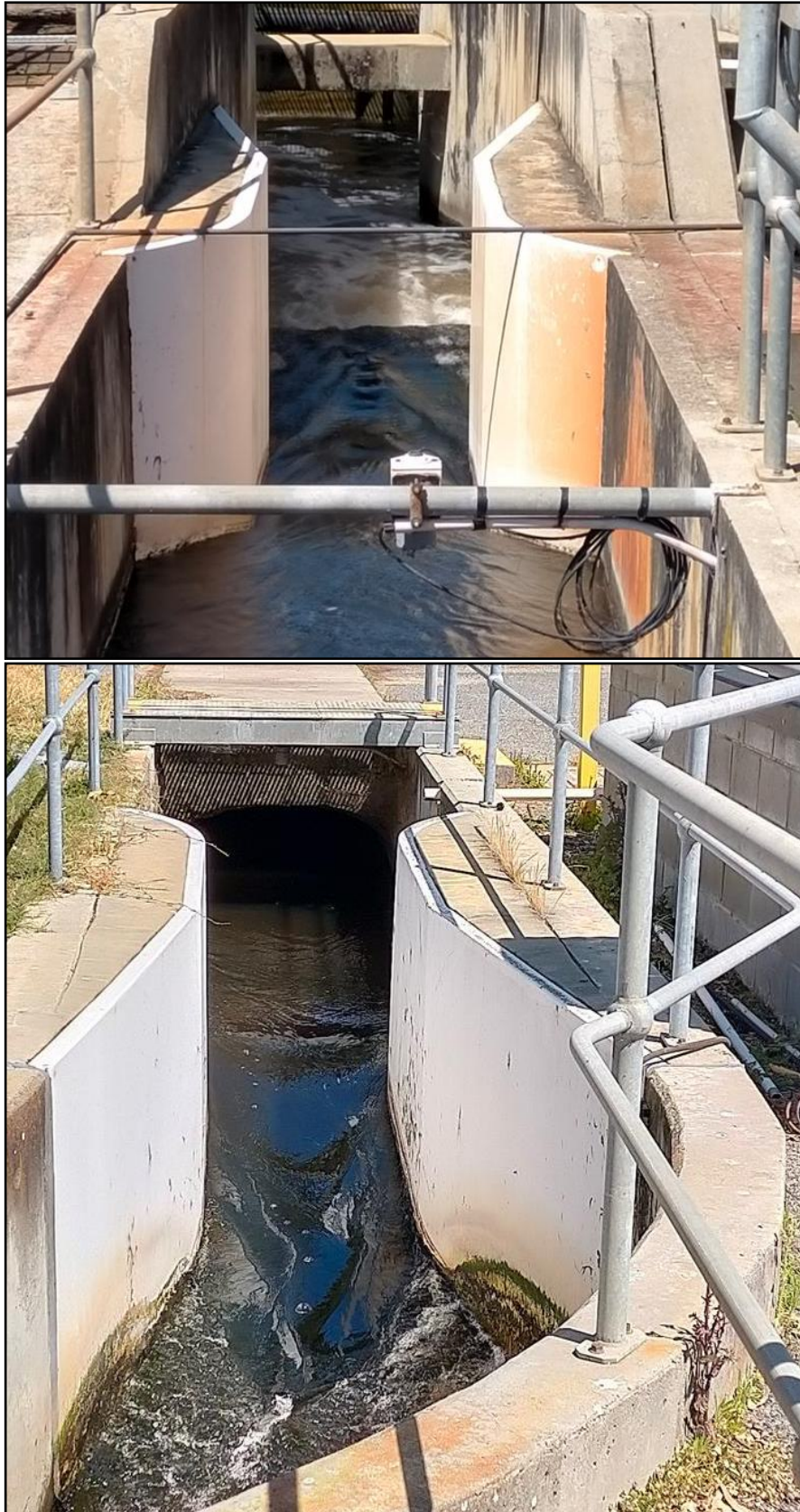
Figure 24: Flumes used to measure final effluent, note the free discharge downstream on the flume.
