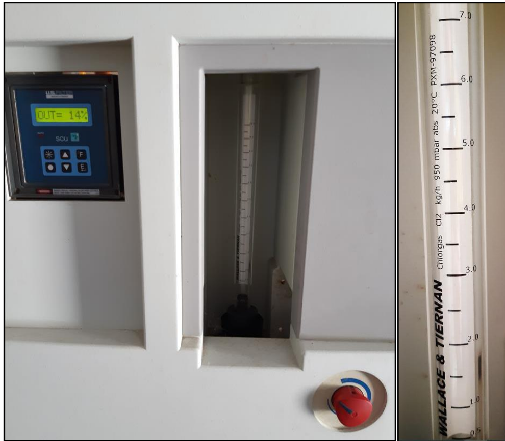
Figure 36: Rotameter on a Chlorine gas vacuum system.
