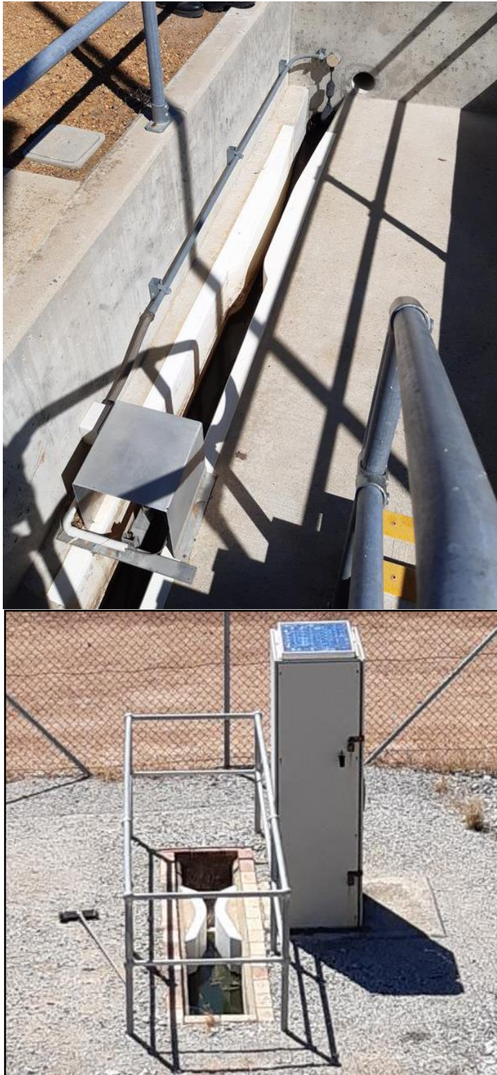
Figure 25: Flumes: Top - treatment plant inflow at Kojonup, Bottom - treated water from ponds to storage dam at Toodyay.
