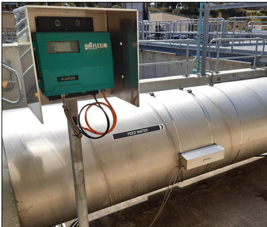
Figure 20: Strap-on ultrasonic flow meter on the feed water line to AWRP.
