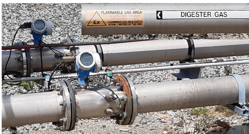
Figure 34: Multi-path ultrasonic flow meter on line to biogas burners at Beenyup WRRF
