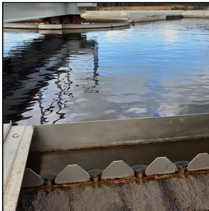
Figure 29: Example of v-notch weir being used as overflow control from a secondary clarifier, note level/flow is not being measured in this instance.
