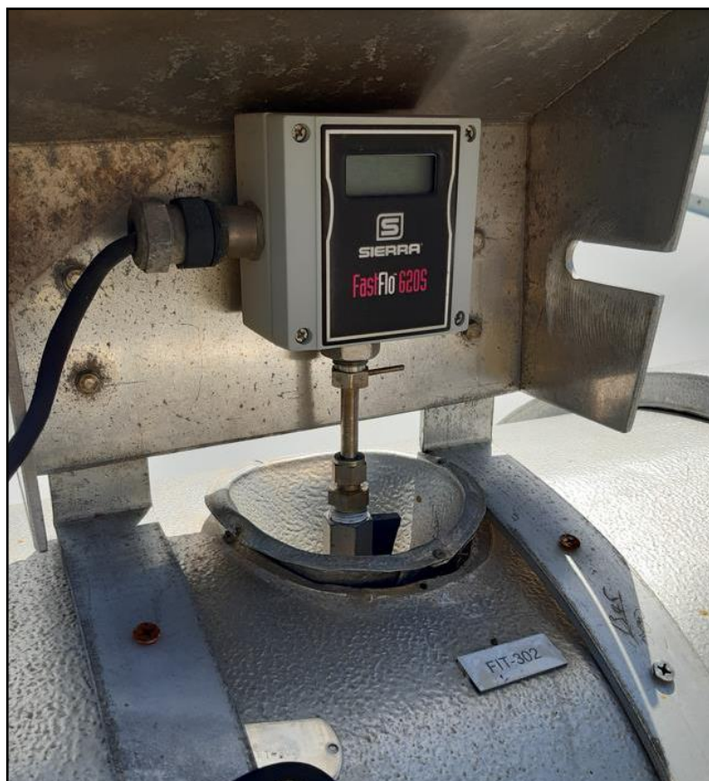
Figure 33: Thermal mass flow meter installed on blower aeration pipework
