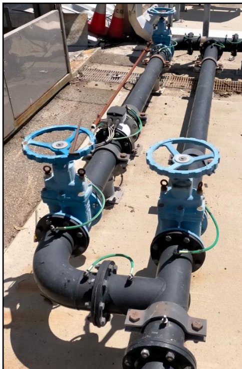
Figure 18: Flow meter installed with a bypass arrangement to facilitate replacement without interrupting flow.
