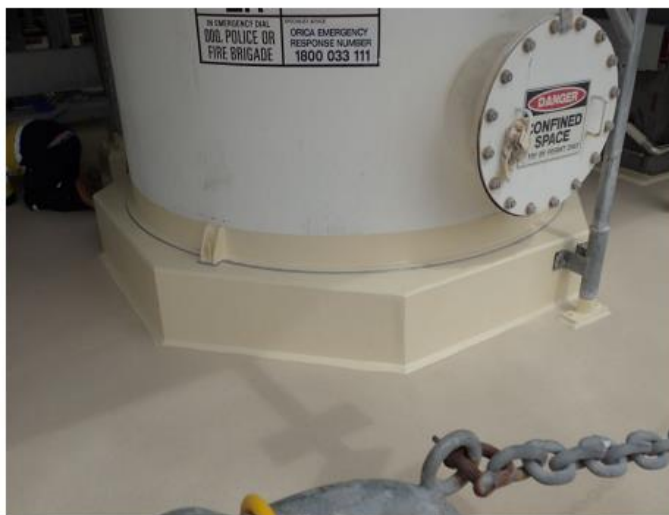
Figure 5 – Example typical coating finish at the interface between concrete and steel/other
