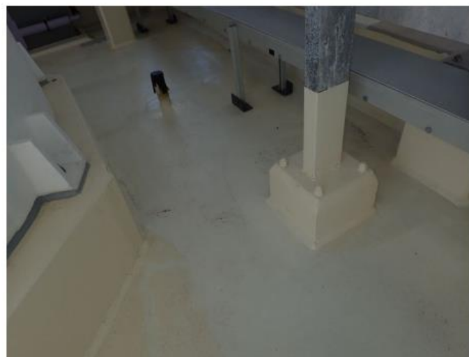
Figure 5 – Example typical coating finish at the interface between concrete and steel/other
