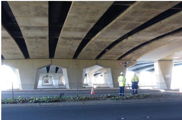
Photo 13a – Pipework and hangers on the underside of the bridge using RPA.
