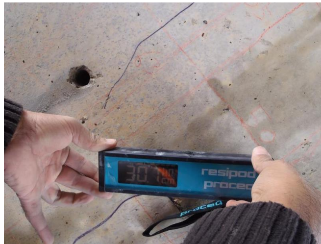
Photo 31 - Concrete Resistivity Meter.
