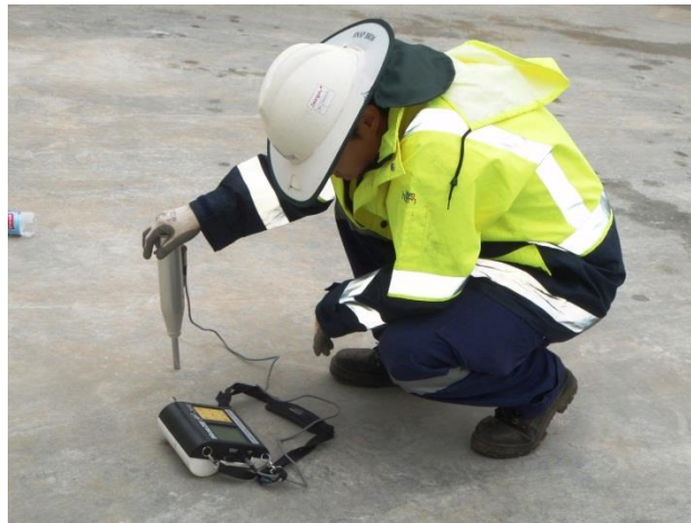
Photo 29 - Schmidt hammer test.
