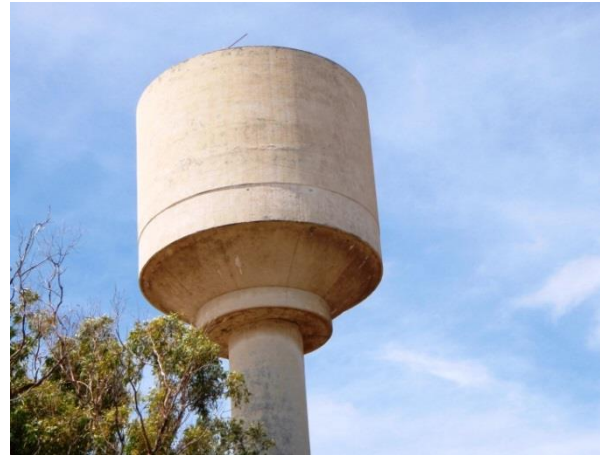
Photo 2 - Elevated concrete potable water tank.
