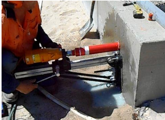
Photo 25 - Concrete coring.
