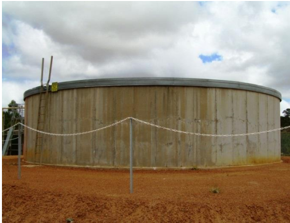
Photo 1 - Ground Level concrete potable water tank.
