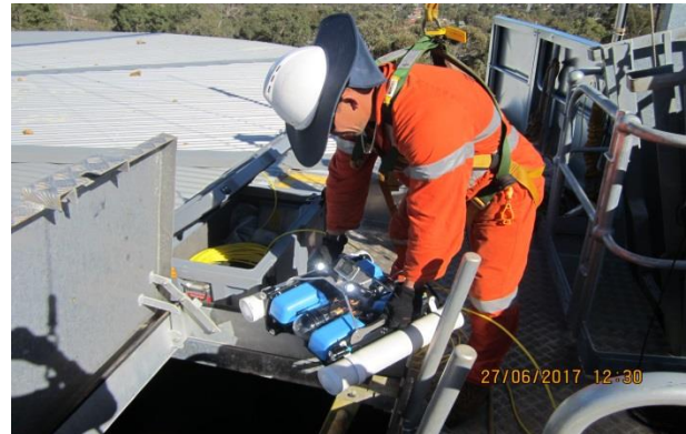
Photo 13 b– Tank inspection by ROV.
