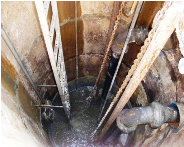
Photo 9 - Sewer wet well.
