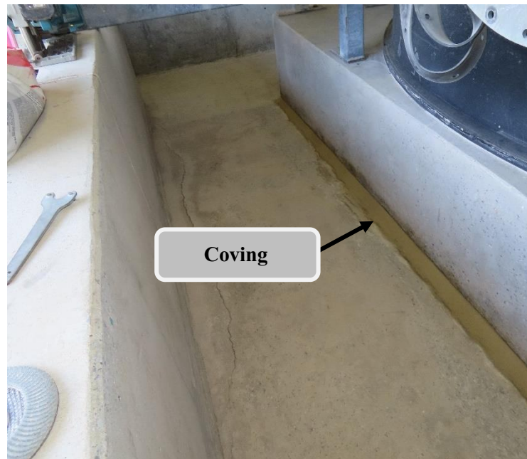
Figure 2 – Example of coving on the floor to wall joint
