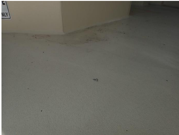
Figure 5 – Full coating on the anti-skid floor
