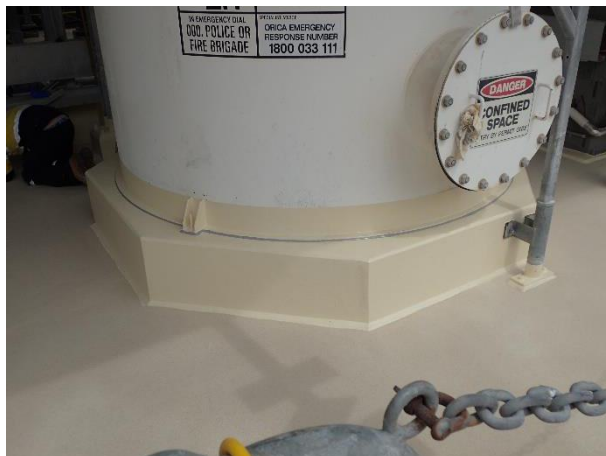
Figure 6 – Typical coating finish at the interface between concrete plinth and tank wall
