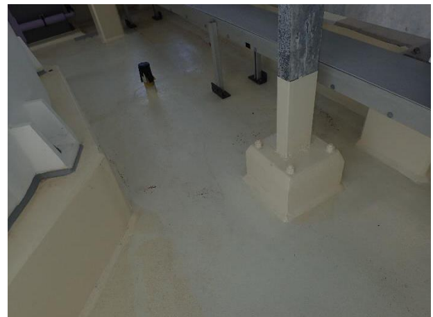
Figure 7 – Typical coating finish at the interface between concrete plinth and pipe supports
