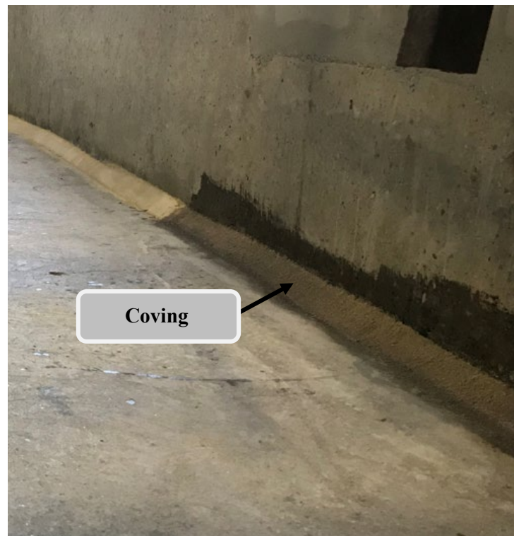
Figure 2 – Coving on the floor to wall joint
