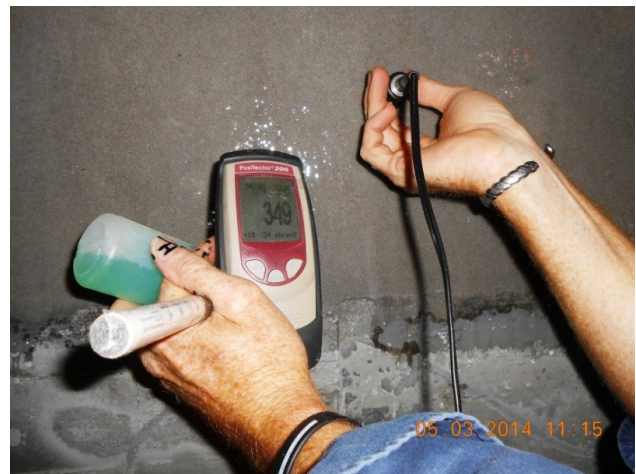
Figure 9 – DFT testing using Positector® gauge
