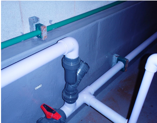
Figure 3 – Full coating on the internals of the concrete wall.
