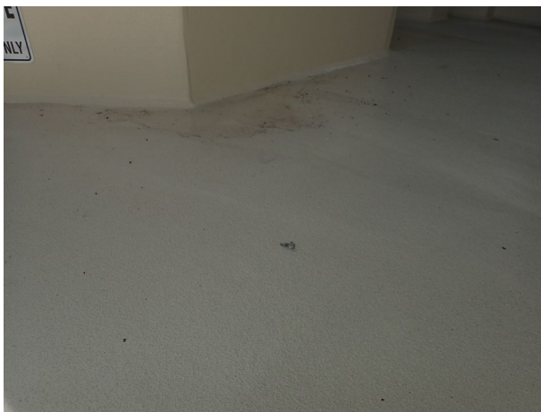
Figure 5 – Full coating on the anti-skid floor
