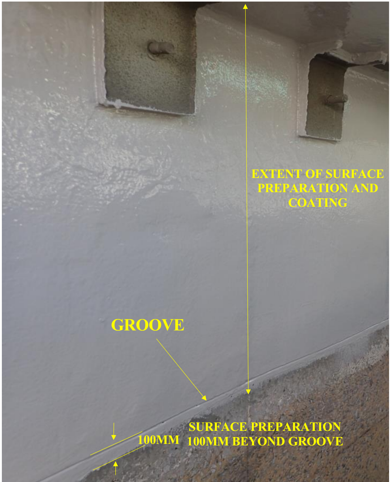
Figure 1 – Termination groove and prepared concrete substrate.
