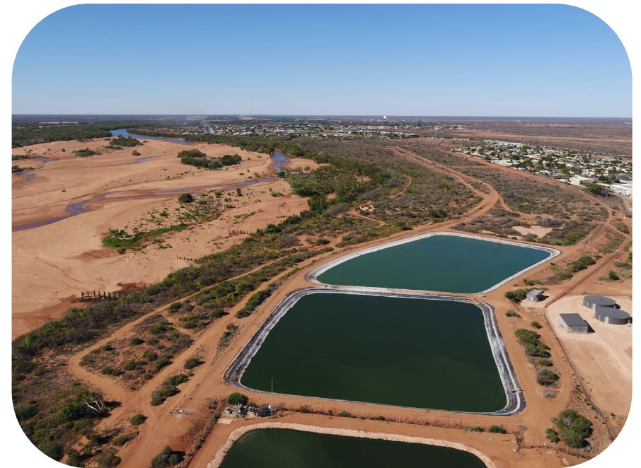
Figure 2: Carnarvon WWTP – wastewater treatment ponds
