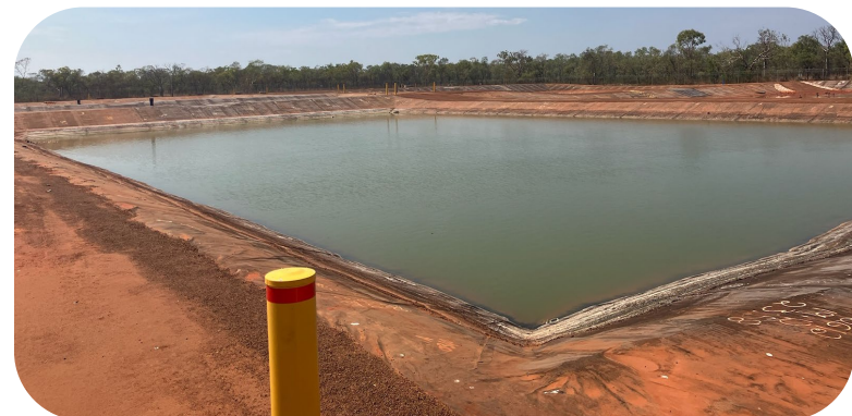
Figure 9: Mowanjum WWTP pond
