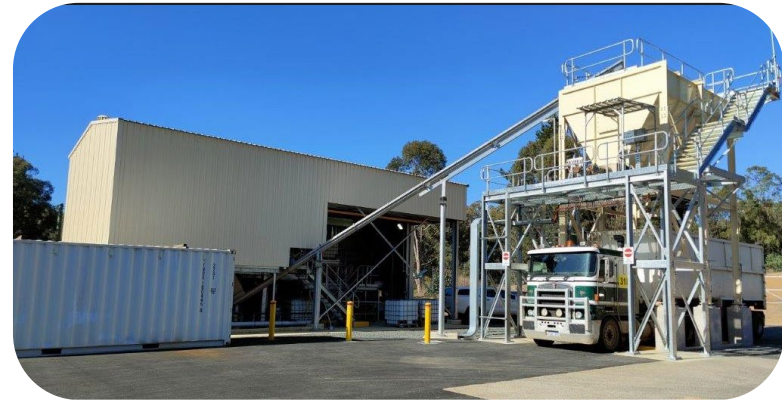
Figure 8: Dewatering building at Collie WWTP
