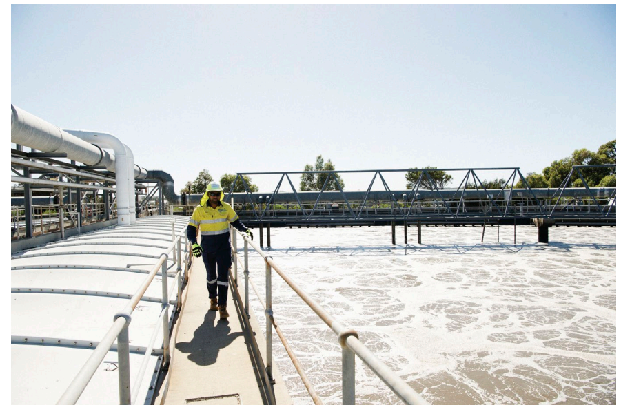
Figure 2: Woodman Point WWTP
