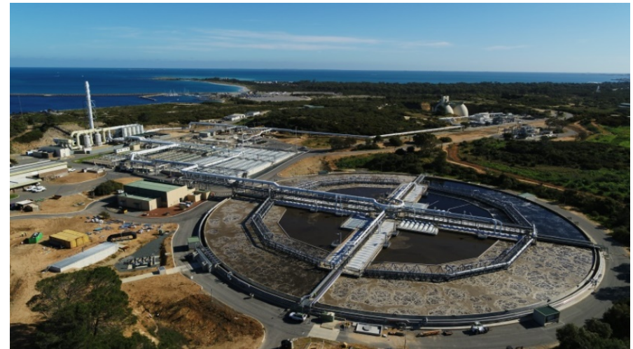
Figure 7: Woodman Point WWTP
